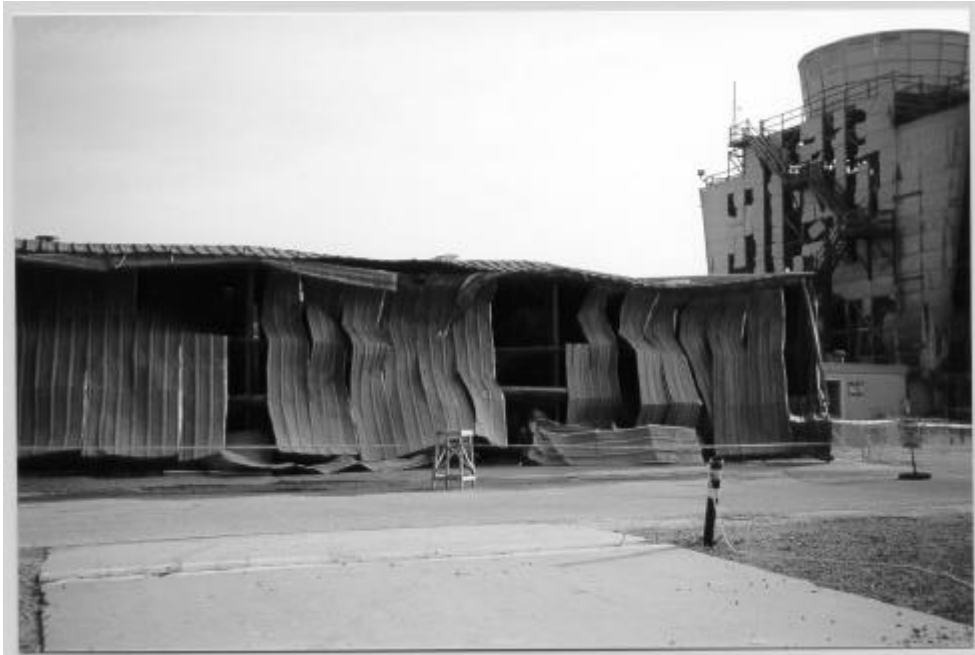
Figure E-7: Photograph of blast damage to buildings and structures in the vicinity of the explosion. Note the buckled metal walls of the storage building in the center and the panels missing from the cooling tower on the right. These buildings were located approximately 500 feet north of the blast center.
