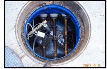
Transition/intermediate sump
