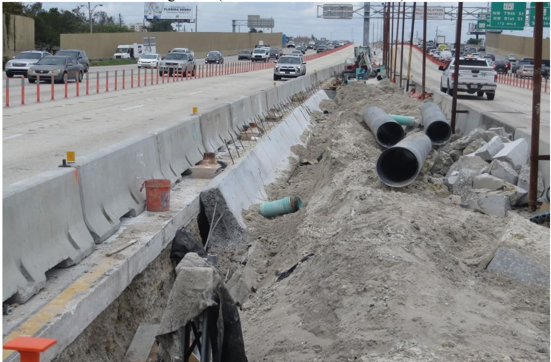
Figure 6 South end of the concrete barrier wall
