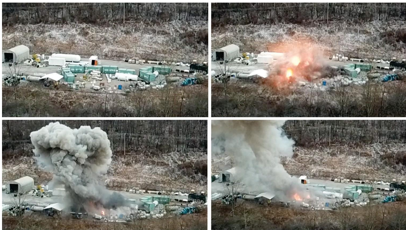
Figure 19. Explosive Venting. These drone video images show the explosive venting used to cut holes in a group of MP vessels to drain the vessels while minimizing risk to people. The bottom right image shows a fire that erupted from flammable liquids that drained from some of the MP vessels. (Credit: MRR).
