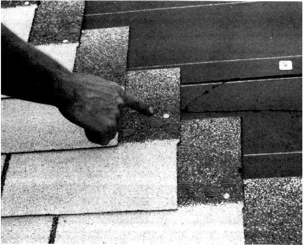
Figure 4. Asphalt shingles nailed too high.
