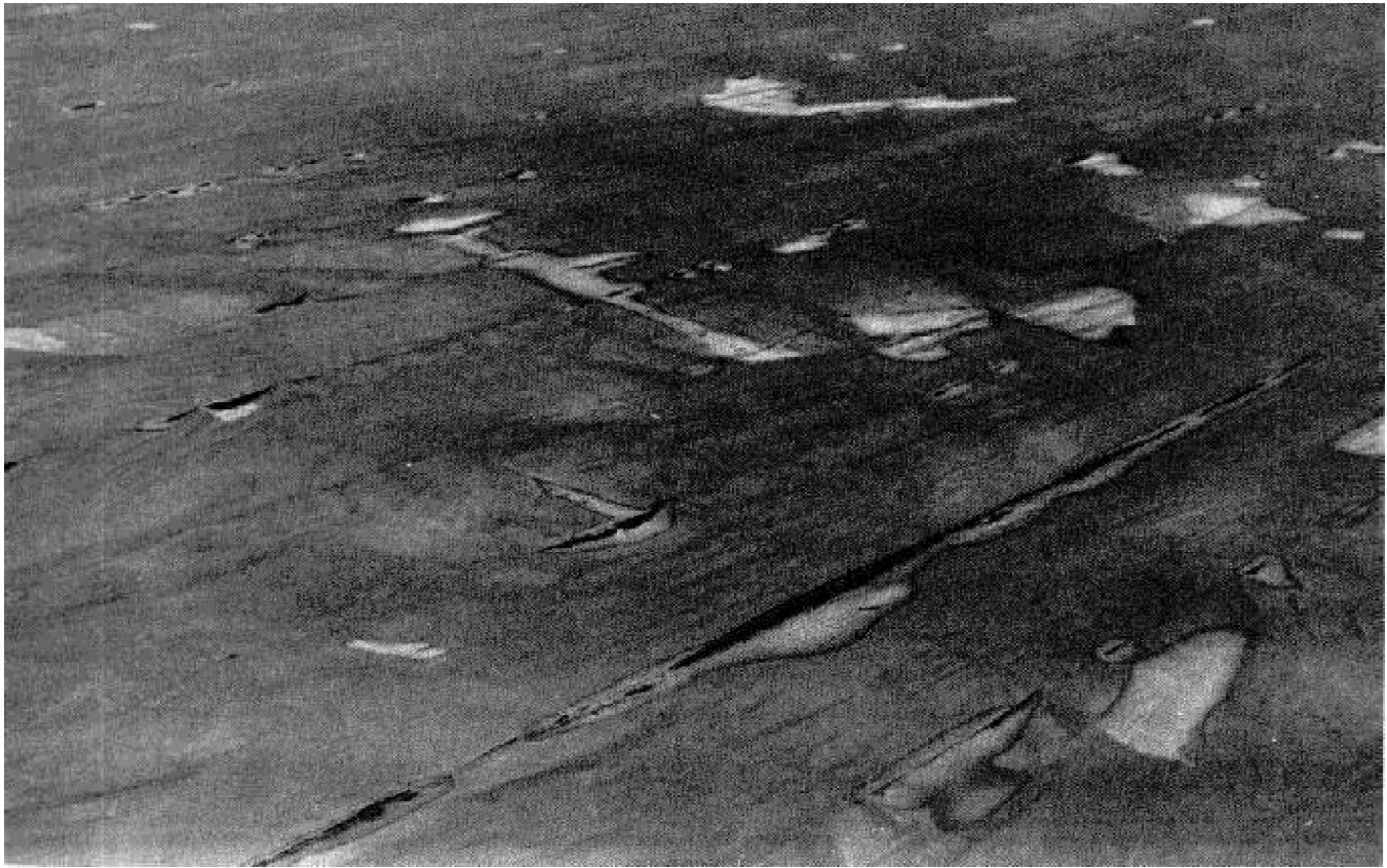
Figure 3. Wrinkles, buckles, lack of adhesion of felts.
