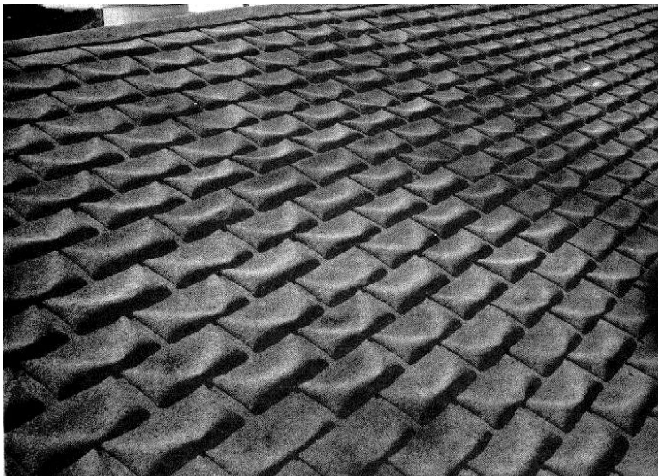
Figure 26. Clawed asphalt strip shingles.
