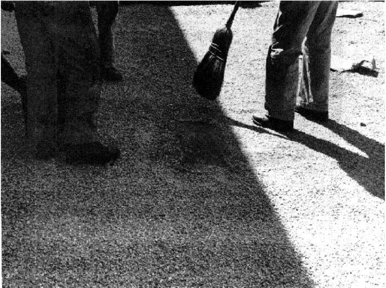
Figure 11. Insufficient bitumen to embed aggregate surfacing.
