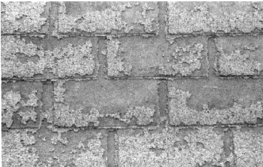
Figure 25. Severe loss of mineral granules and coating asphalt due to weathering.
