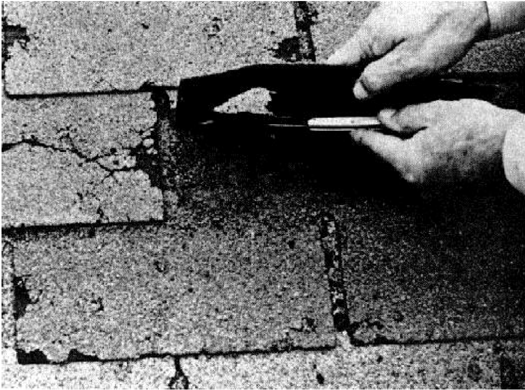
Figure 30. Hail damage showing broken shingles — reroofing mandatory.
