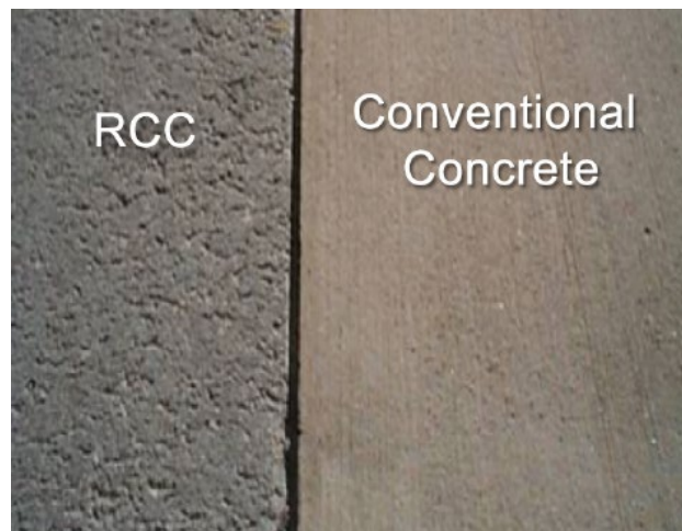
Figure 5. RCC surface texture.
