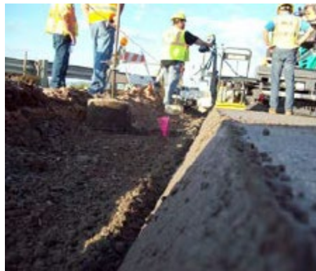
b Angular Cold Joint.
