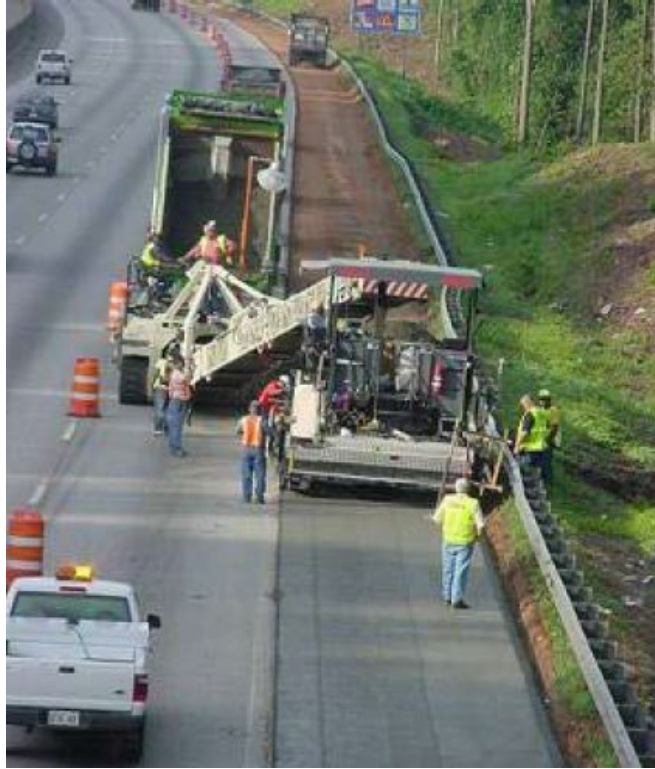
Figure 9. RCC construction.
