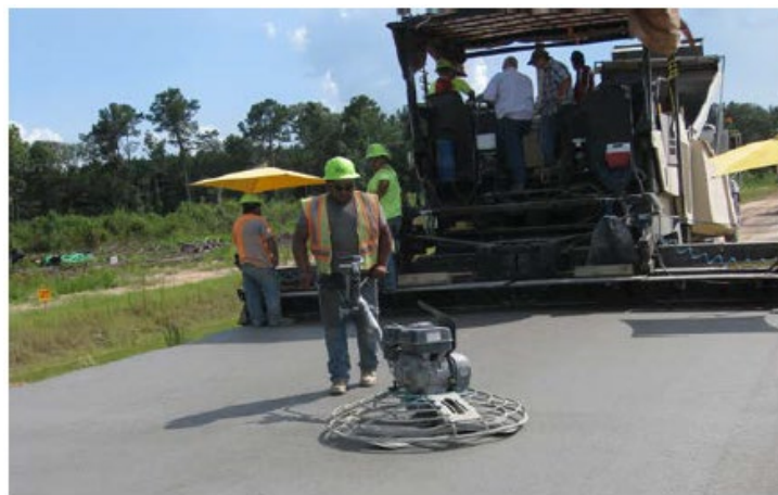
Figure 12. Method to improve upon RCC finished surface.
