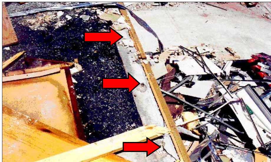
FIGURE 5-22: Attachments of lower plates for wall to hollow core plank using power driven anchors failed when required to carry loads generated by the winds of a moderate tornado vortex. This motel was located in Midwest City, Oklahoma.
