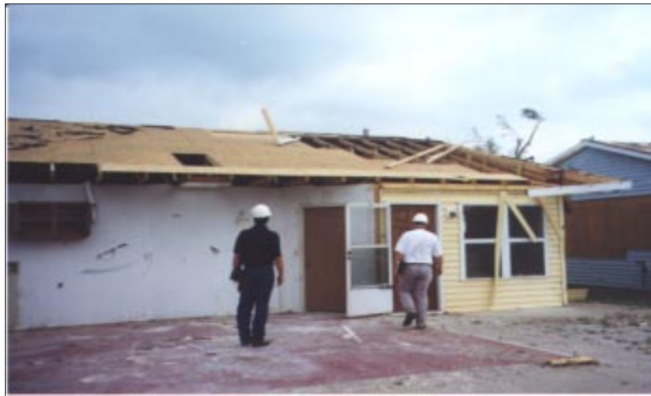
FIGURE 4-4: Although roof sheathing was lost at this Wichita, Kansas, home code requirements of staggering joints in sheathing applications was observed. This house experienced inflow winds from a severe tornado.
