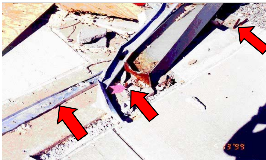
FIGURE 5-6: Attachment of columns to foundation and attachment of wall bottom plates to concrete slab. Regional outlet mall, Stroud, Oklahoma, hit by moderate tornado vortex.
