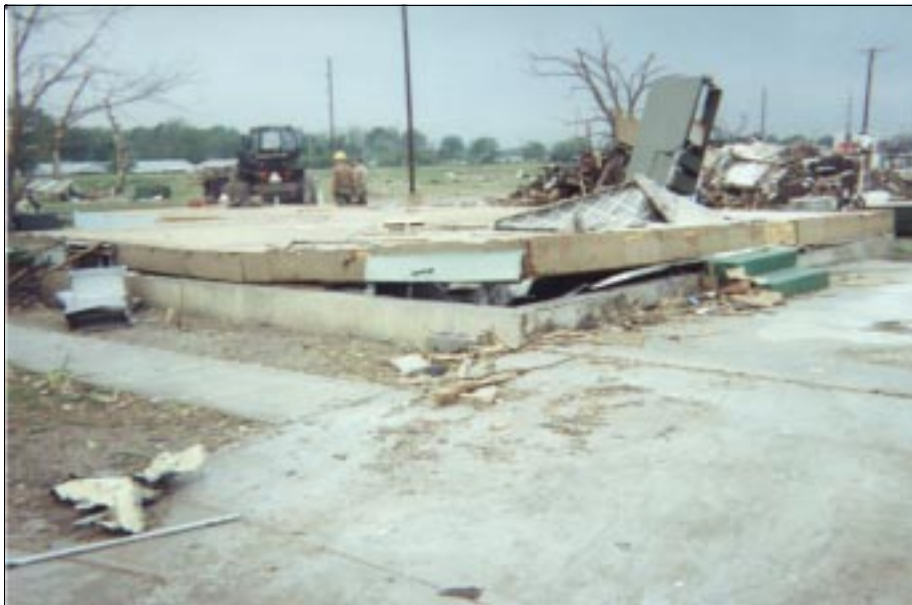
FIGURE 3-3: Wind uplift acting on this house in Haysville, Kansas, resulted in this corner of the building being lifted off its foundation.
