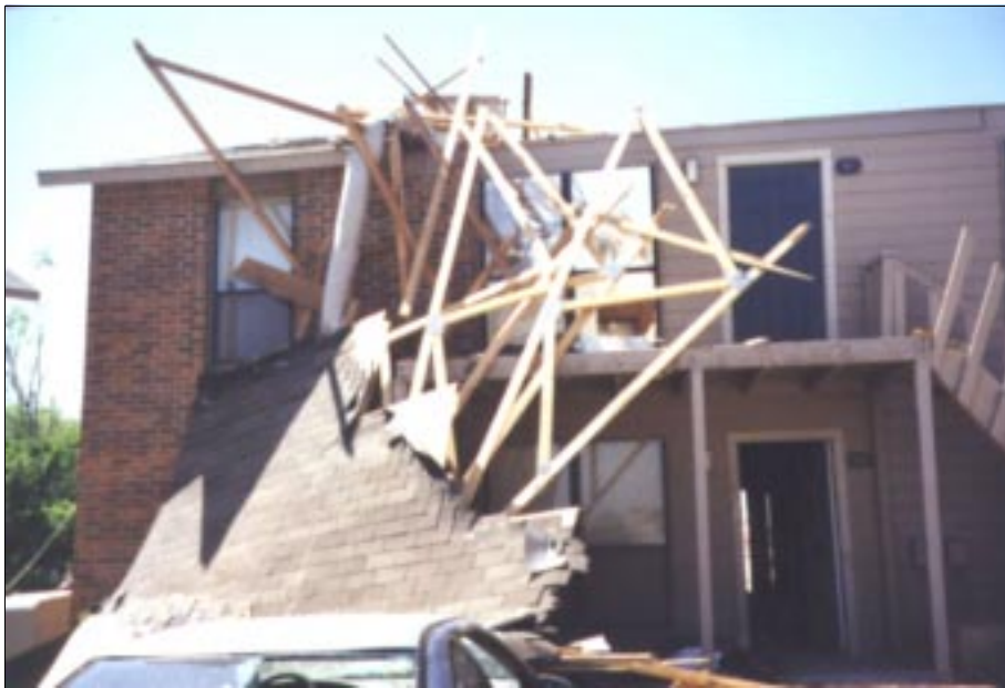
FIGURE 3-13: These trusses and roof covering (still attached to the roof sheathing) was displaced by the winds of a violent tornado and are capable of becoming large, windborne missiles.
