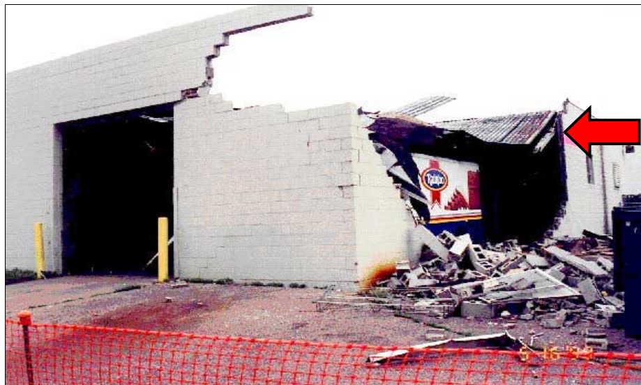
FIGURE 5-26: Failure of roof and walls on structure due to increased loads caused by initial failure of garage door, Wichita, Kansas.
