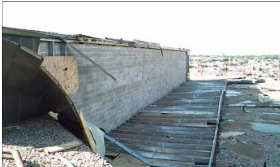
FIGURE 5-24: This metal-clad wall covering collapsed and in other areas it was blown completely away.
