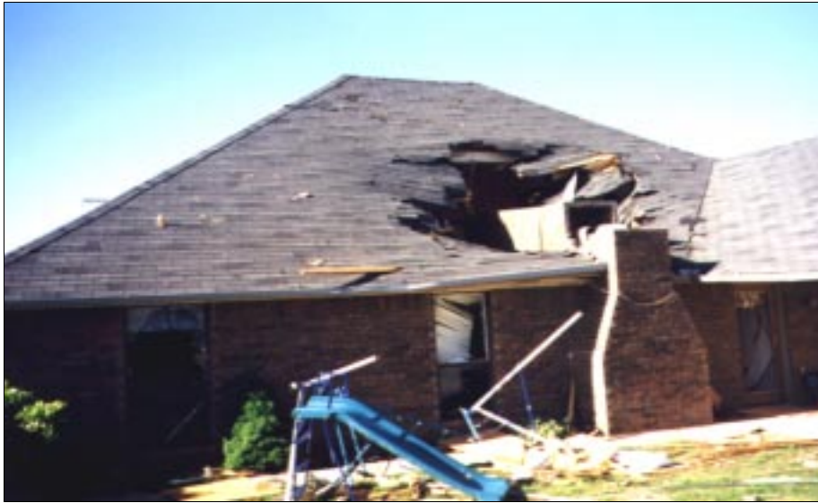
FIGURE 4-42: Failure of brick chimney onto top of home located along the periphery of a violent tornado, Moore, Oklahoma.
