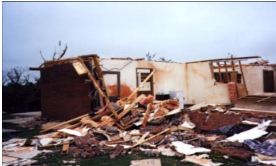
FIGURE 4-30: Failure of brick masonry veneer construction. The vortex of the severe tornado that caused the winds at this site passed approximately 30 feet from this building in Bridge Creek, Oklahoma.
