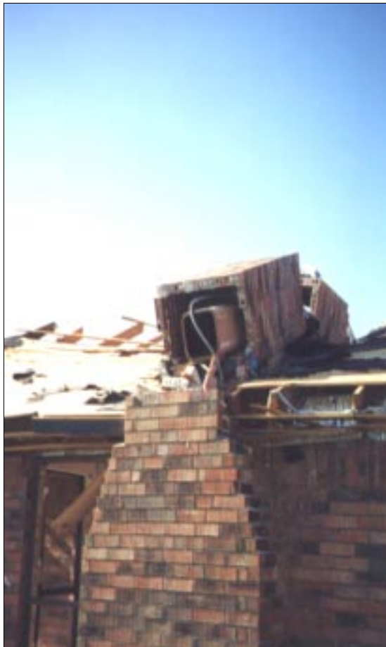
FIGURE 4-41: Close-up view brick chimney failure in Figure 4-40.
