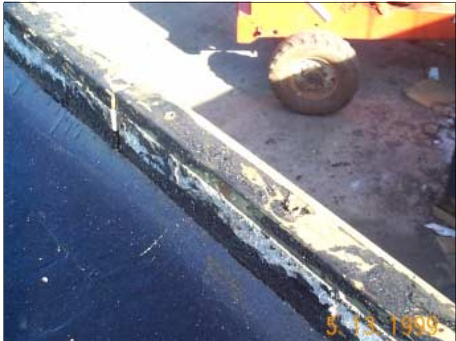
Figure 5.23: Nailer at the roof of the hospital in Stroud, Oklahoma. The roof surface in this photo was replaced prior to this photo, but the same nailer was used again.
