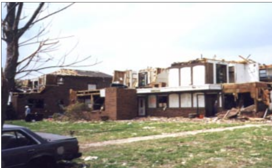
FIGURE 4-43: Failure of masonry veneer.
