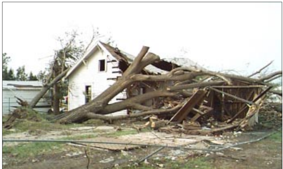
FIGURE 3-22: This building was on the periphery of a violent tornado damage area in Haysville, Kansas. One large tree fell near the corner of the house and collapsed a large portion of the roof and the corner walls. A smaller tree caused minor damage on the other corner of the house.
