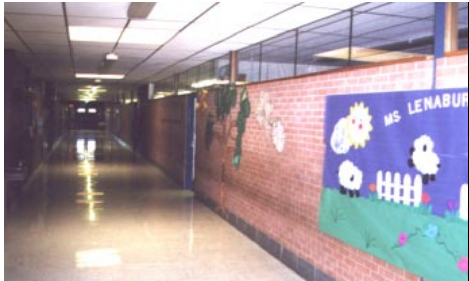
FIGURE 6-31: Northmoor Elementary place of refuge, Moore, Oklahoma - double loaded corridor with clerestory windows. This corridor offers little protection from a violent tornado as shown in a school of similar design in Figure 6-32.
