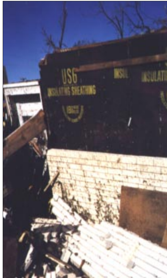
FIGURE 4-39: Failure of masonry veneer wall of home located along the periphery of a violent tornado, Del City, Oklahoma.
