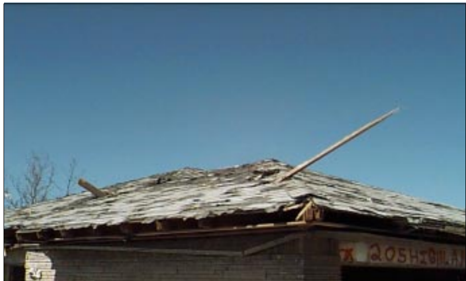
FIGURE 3-26: This house was on the periphery of a violent tornado damage area in Moore, Oklahoma. Two large missiles struck this area of the roof.
