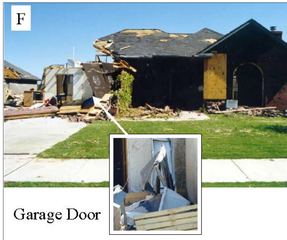
FIGURE 4-22: Garage door failure possibly resulting in the localized partial roof failure on the left side of this home located in Moore, Oklahoma.
