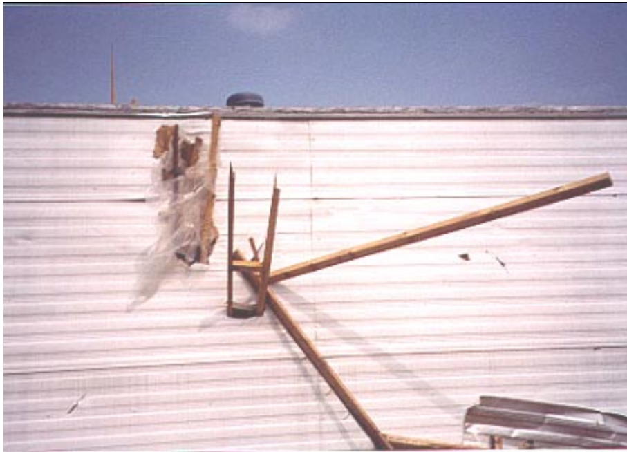
FIGURE 3-12 These medium sized missiles struck and remained embedded within this manufactured home in Wichita, Kansas.
