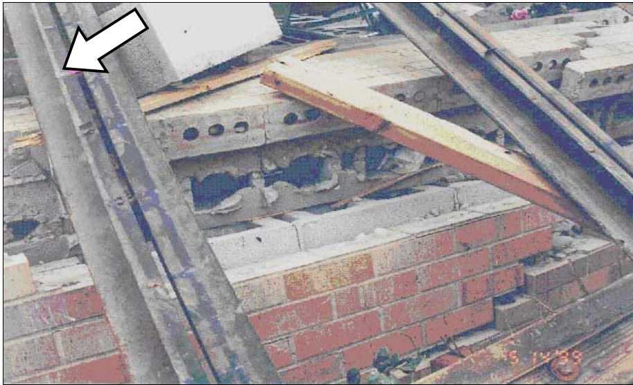
FIGURE 5-4: Failed structure showing broken deck welds, and no effective vertical reinforcement. Kelly Elementary School, Moore, Oklahoma, hit by vortex of violent tornado.
