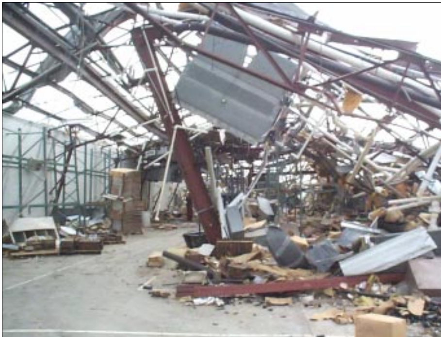
Figure 3-10: The vortex of a violent tornado passed within 100 yards of this plastics manufacturing plant in the City of Haysville, Kansas. The wind forces caused the failure of its primary structural system: a steel frame with masonry infill walls.
