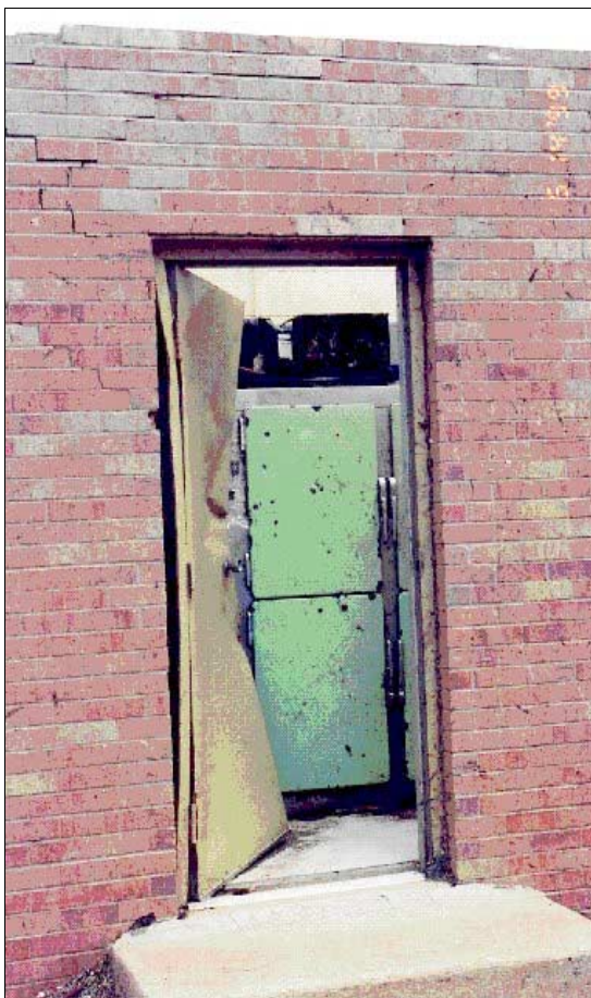
FIGURE 5-28: Damaged door most likely opened by impact with heavy object. Kelly Elementary School, Moore, Oklahoma.
