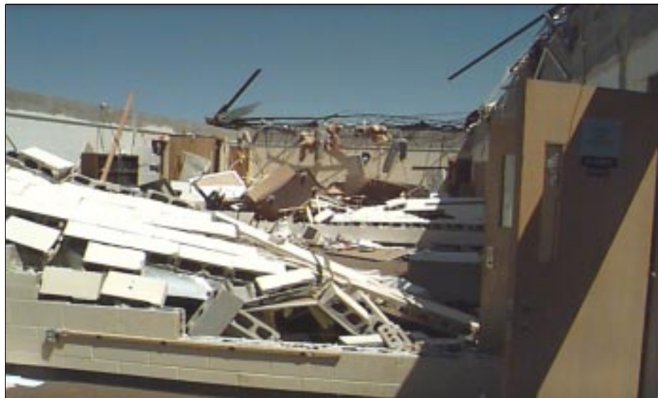
FIGURE 6-35: The non-reinforced interior CMU walls in this area of Kelly Elementary collapsed after the roof system was removed by vortex winds of a violent tornado.
