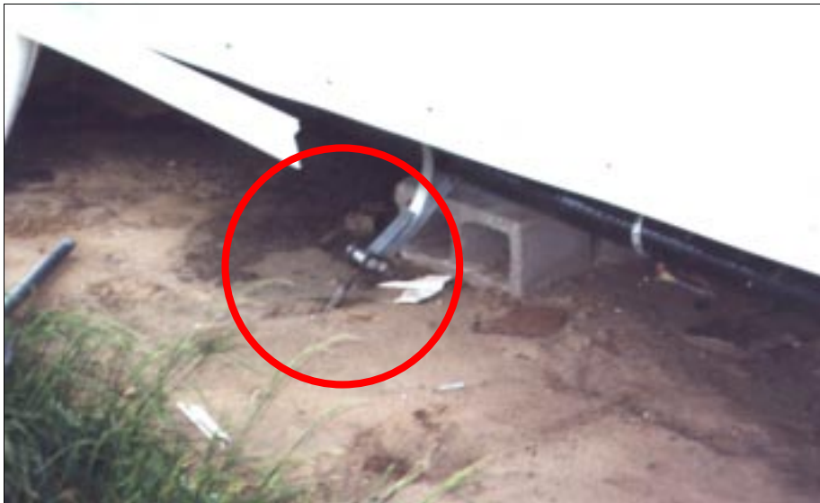
Figure 4-52: Anchor of manufactured home bent and pulled up from soil. This home in Wichita, Kansas, was located within the inflow area of a severe tornado.
