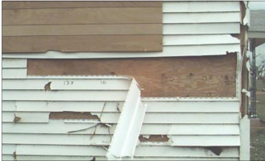
FIGURE 4-17: Some pieces of vinyl siding were blown off and in other areas the siding was torn away by missiles. The home was located along the periphery of a violent tornado in Mullhall, Oklahoma.
