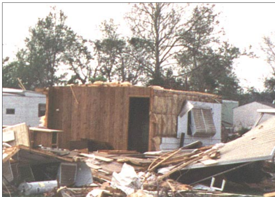
Figure 4-54: Roof and wall damage experienced due to inadequate resistance to lateral and uplift wind forces associated with straight inflow winds of a moderate tornado, Wichita, Kansas.
