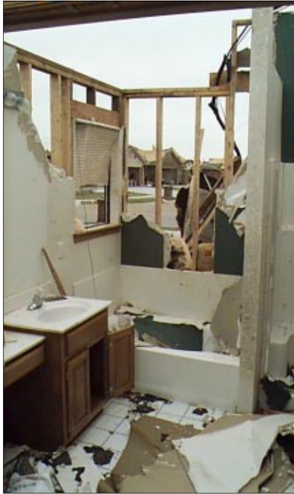
FIGURE 6-26: This bathroom was on an exterior wall and had a window. It was not a safe refuge.
