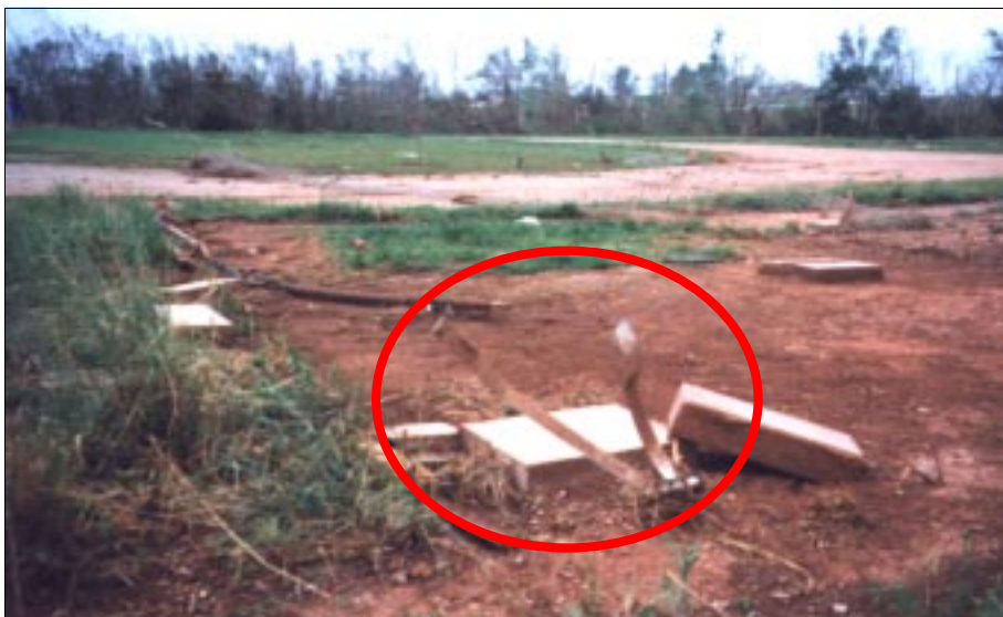
FIGURE 4-49: Failed straps at the anchorage of a manufactured home in Bridge Creek, Oklahoma. This site was 300-400 feet from a violent tornado vortex.
