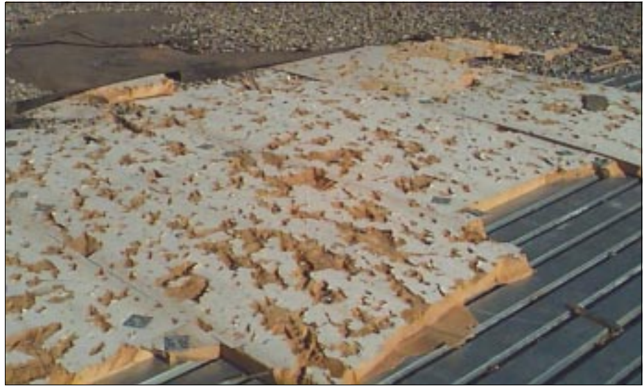
FIGURE 3-25: Close-up view of roof insulation boards (the boards are 4-ft by 8-ft) at Westmoore High School. This roof is approximately 35 feet above grade. Some of the missiles only caused superficial damage to the insulation, but several others had sufficient force to make large gouges in the insulation.
