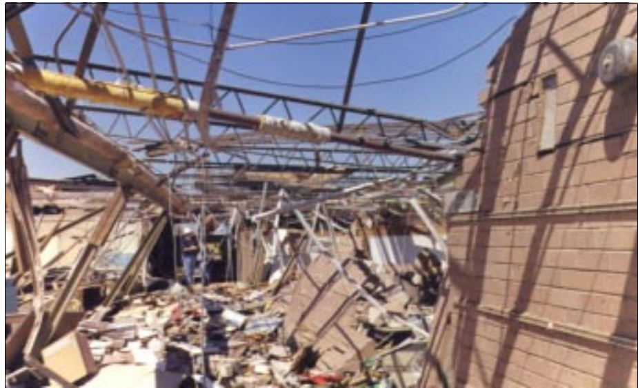
FIGURE 6-32: Kelly Elementary School, Moore, Oklahoma, place of refuge - double loaded corridor with clerestory windows. These interior corridor walls had brick masonry up to a height of approximately 7 feet. Glass extended from the top of the masonry to the top of the wall.
