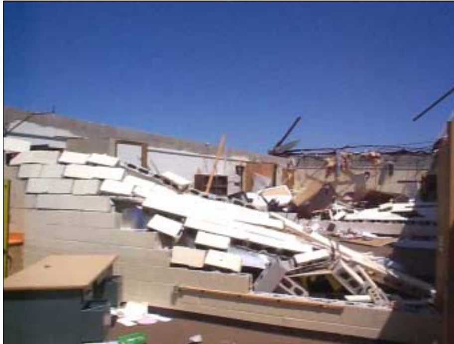
Figure 5-20: Damage to interior and exterior unreinforced masonry walls when bond beam failed at Kelly Elementary School in Moore, Oklahoma. The school was struck by the vortex of a violent tornado.
