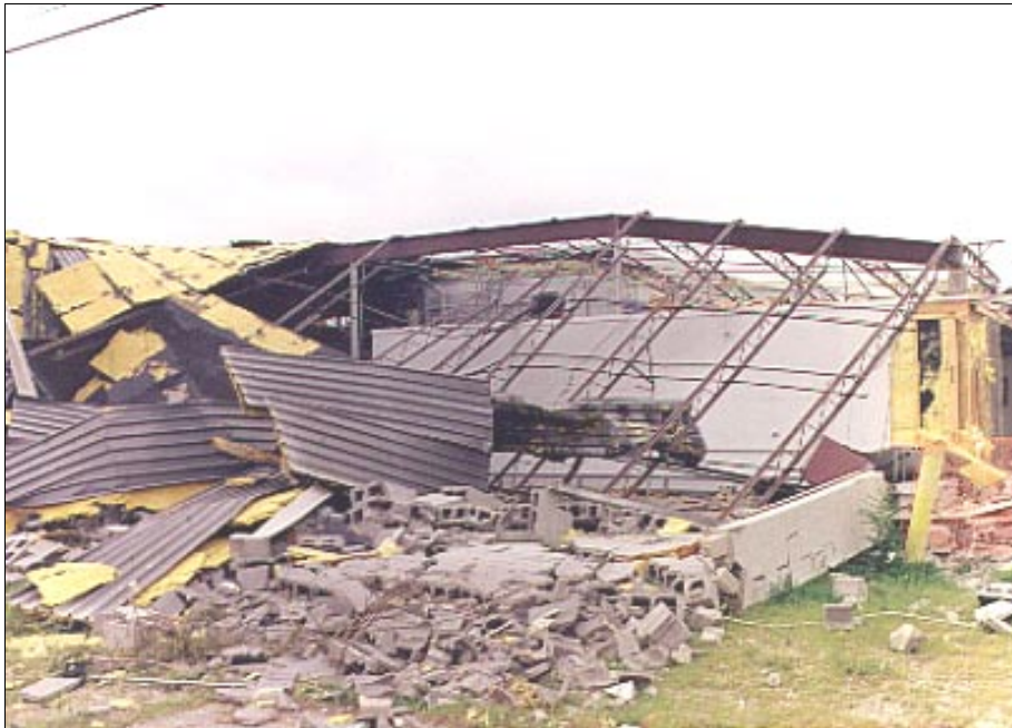
Figure 3-9: This URM wall failed when inflow winds from a severe tornado acted on this building in Wichita, Kansas.
