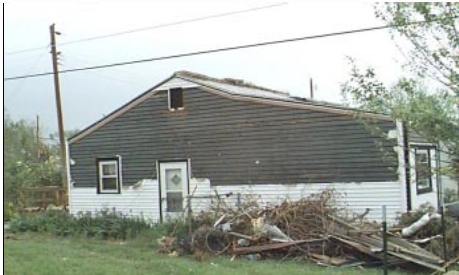
FIGURE 4-16: The vinyl (white) that was installed over wood siding experienced damage; however, the wood siding was undamaged. The home was located along the periphery of a violent tornado in Wichita, Kansas.
