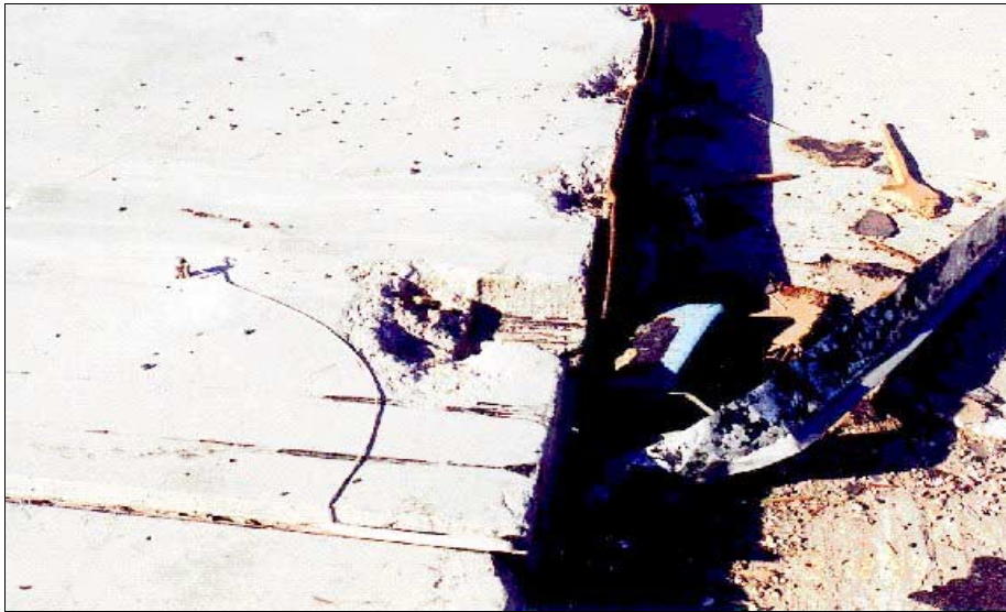
FIGURE 5-17: Top of failed tilt-up wall.
