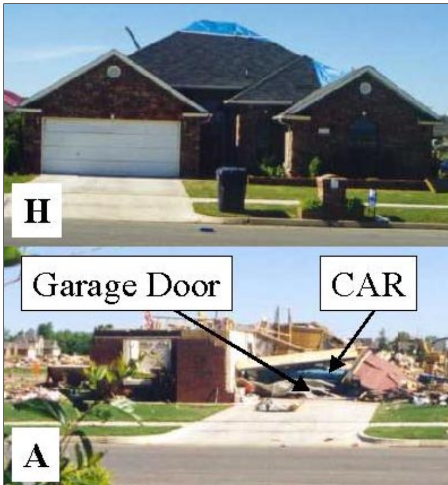
FIGURE 4-20: Home in Moore, Oklahoma, with partial roof loss (H) vs. home with total roof loss due to garage door failure (A) under positive pressure.
