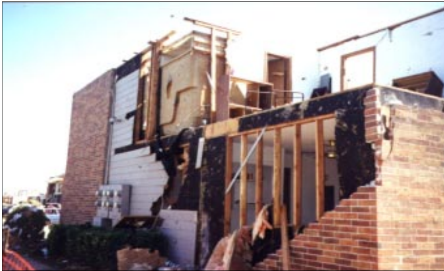
FIGURE 4-11: Stud-wall and sole-plate-to-floor failure on a second story wall. This multi-family residence in Wichita, Kansas, was located approximately a few hundred feet from the vortex of a violent tornado and was exposed to inflow winds.
