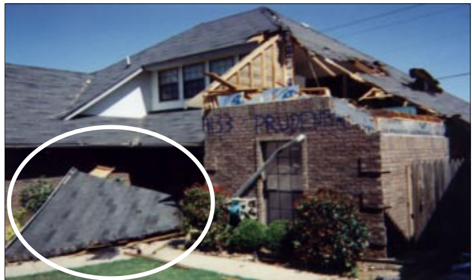
FIGURE 3-5: Failure of hip roof due to internal pressures and leeward wind forces acting together. This house, which was exposed to inflow winds of a violent tornado, was located in a suburb of Oklahoma City, Oklahoma.
