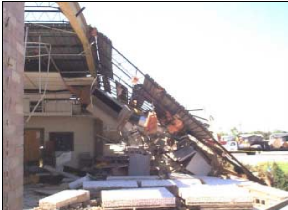
FIGURE 5-13: Collapsed roof structure and exterior at Kelly Elementary School in Moore, Oklahoma struck by the vortex of a violent tornado.
