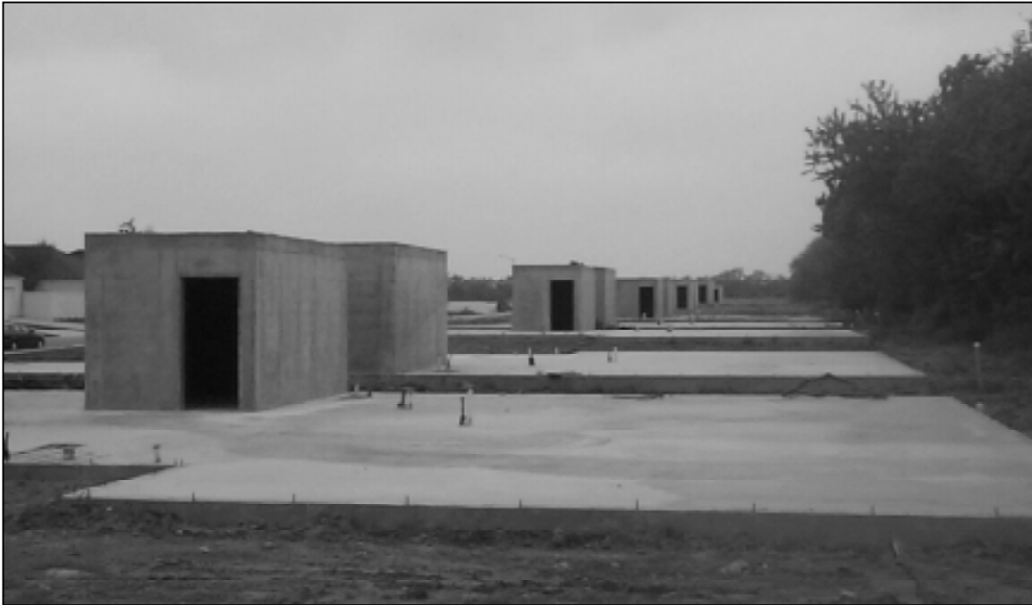
Tornado shelters under construction in the Country Club Courts subdivision by The Core Inc., Wichita, Kansas
