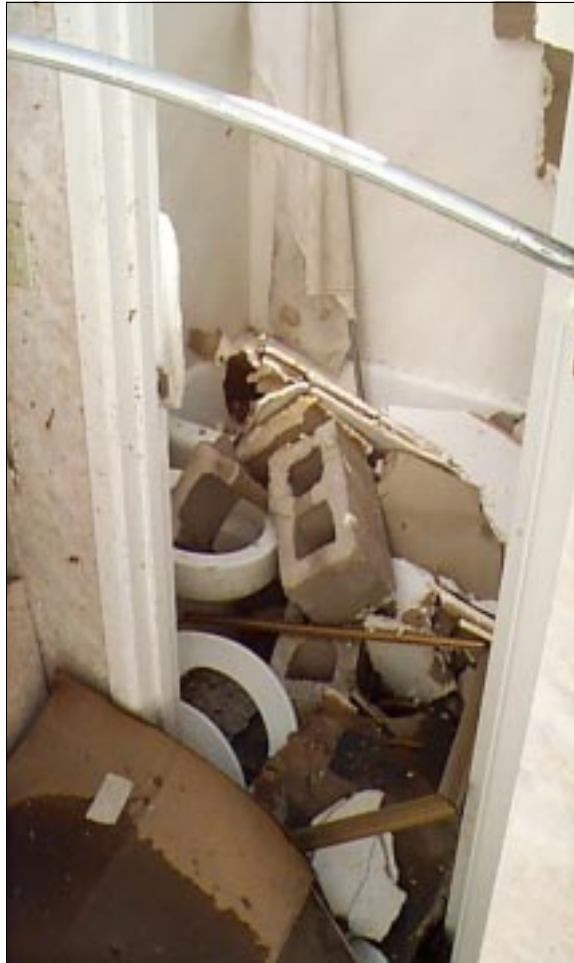
FIGURE 6-36: The roof and ceiling over this interior bathroom blew off. CMU from a firewall a few feet away blew into the bathroom, which was located on a motel's second floor in Mid West City, Oklahoma. This bathroom was not a safe refuge when impacted by the vortex of a severe tornado.
