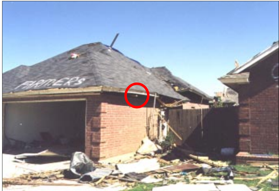
FIGURE 4-21: A 2x4 member extends out of the gap that runs the length of this garage wall between the top of the wall and the roof framing
