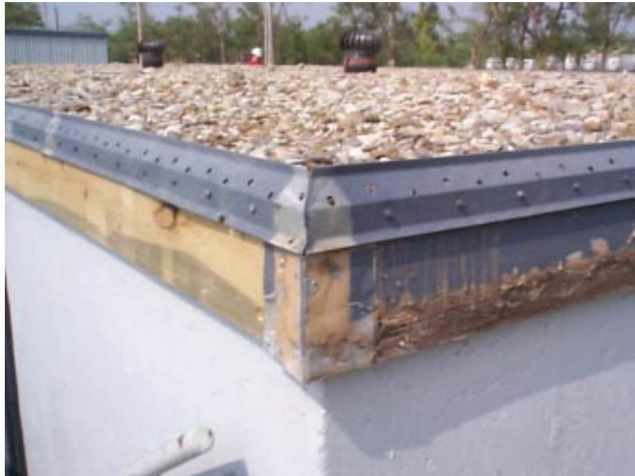
FIGURE 6-15: Ballast roof covering on a community shelter in Wichita, Kansas was a potential source of deadly windborne missiles to those seeking to access the shelter.
