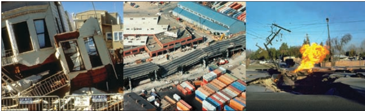
Loma Prieta Earthquake, CA, October 18, 1989 (left to right) – The first story of this three-story apartment building located in the Marina District of San Francisco failed when ground shaking caused liquefaction of the soil on which the structure was built. (D. Perkins, U.S. Geological Survey) Fifty-one spans of this double-decker freeway collapsed in Oakland, killing 41 motorists. (E.V. Leyendecker, U.S. Geological Survey) Northridge Earthquake, CA, January 17, 1994 – A broken gas line on Balboa Boulevard in Los Angeles caused this fire. (M. Rymer, U.S. Geological Survey)
