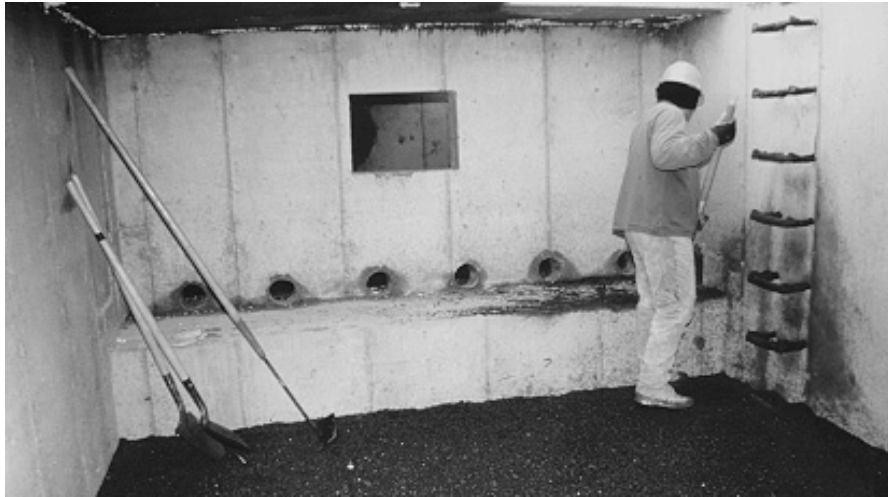
VIEW OF THE INSIDE OF A SAND FILTER SIMILAR TO THE ONE INSTALLED AT DUKE STREET SQUARE
