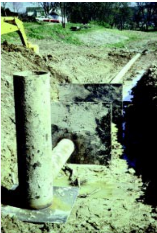
Figure 22 Drop-inlet pipe spillway with antiseep collar
