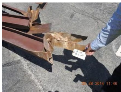
Fig. 35 – Joint 1 – East truss
