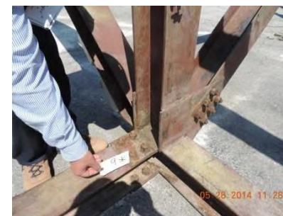
Fig. 60 – Joint 9 – West interior
