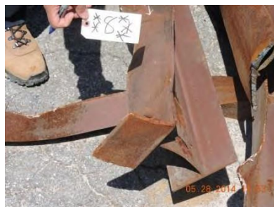
Fig. 51 – Joint 8 – West truss
