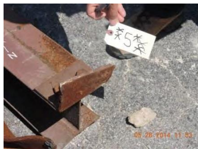
Fig. 48 – Joint 5 – West truss
