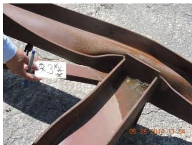
Fig. 46 - Joint 3 – West truss
