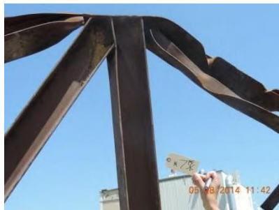
Fig. 32 – Joint 7 – South truss
