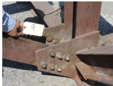
Fig. 74 – Joint 9 – South interior
