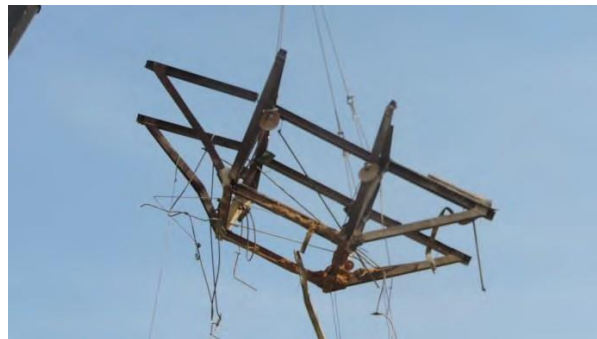
Fig. 105 Interior trusses being retrieved
