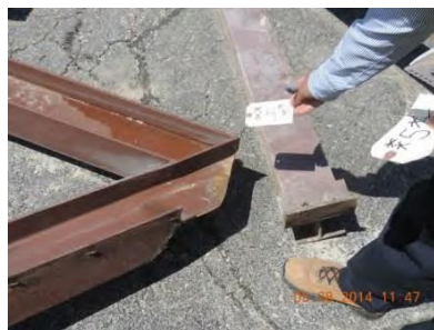
Fig. 38 – Joint 4 – East truss
