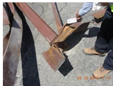
Fig. 36 – Joint 2 – East truss
