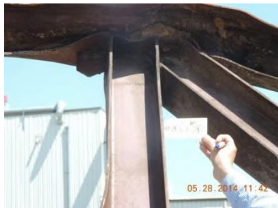
Fig. 31 – Joint 6 – South truss
