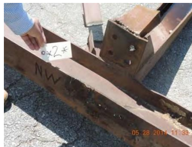
Fig. 17 – Joint 2 – North truss
