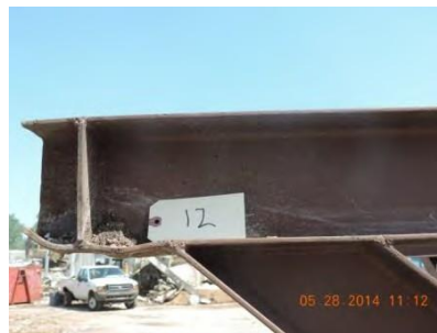
Fig. 77 – Joint 12 – South interior
