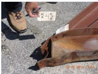
Fig. 47 – Joint 4 – West truss
