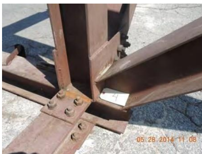
Fig. 67 – Joint 4 – North interior
