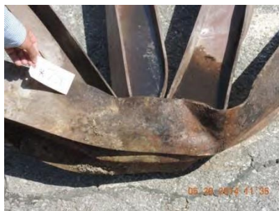
Fig. 22 – Joint 7 – North truss
