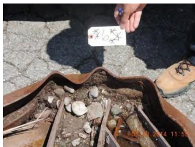
Fig. 49 – Joint 6 – West truss
