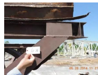
Fig. 57 – Joint 6 – East interior
