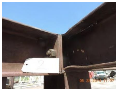
Fig. 65 – Joint 2 – North interior
