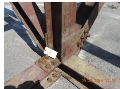
Fig. 66 – Joint 3 – North interior
