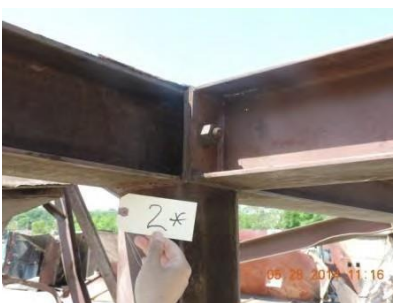
Fig. 53 – Joint 2 – East interior
