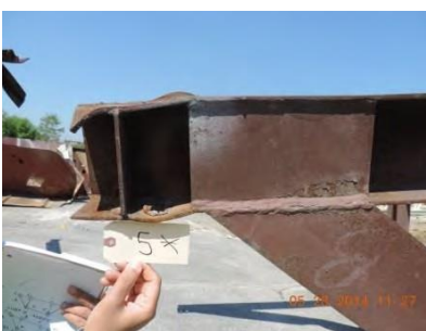
Fig. 56 – Joint 5 – East interior
