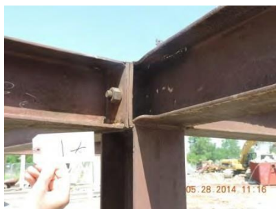
Fig. 52 – Joint 1 – East interior
