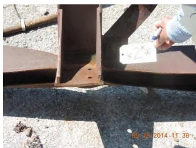
Fig. 26 – Joint 2 – South truss
