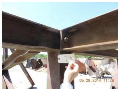
Fig. 58 – Joint 7 – West interior
