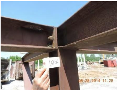
Fig. 61 – Joint 10 – West interior
