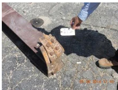
Fig. 34 – Joint 1 – East truss
