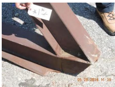
Fig. 25 – Joint 1 – South truss
