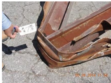
Fig. 42 – Joint 7 – East truss
