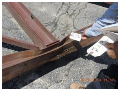
Fig. 37 – Joint 3 – East truss
