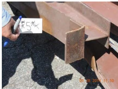
Fig. 40 – Joint 5 – East truss
