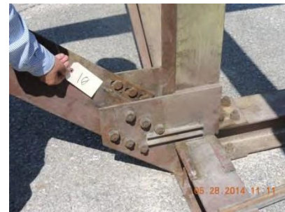
Fig. 75 – Joint 10 – South interior
