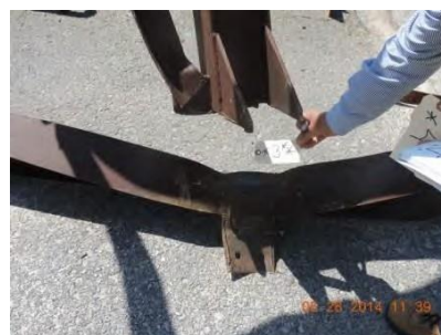
Fig. 27 – Joint 3 – South truss
