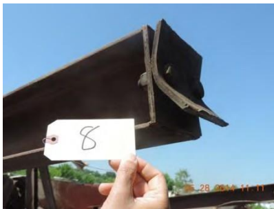
Fig. 73 – Joint 8 – South interior
