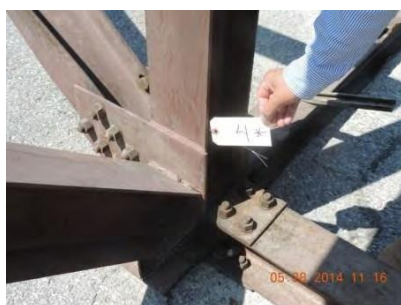
Fig. 55 – Joint 4 – East interior
