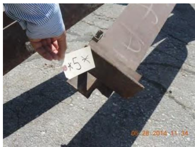
Fig. 20 – Joint 5 – North truss
