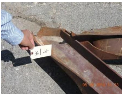
Fig. 16 – Joint 1 – North truss
