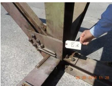
Fig. 59 – Joint 8 – West interior
