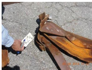
Fig. 45 – Joint 2 – West truss
