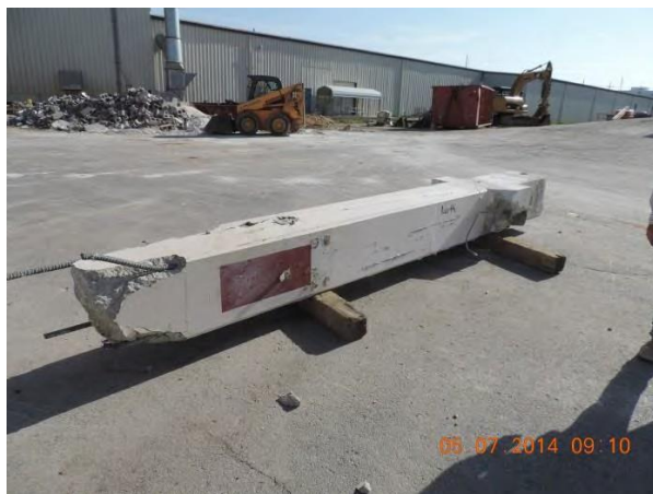
Fig. 102 NE corner column showing inadequate lap splice
