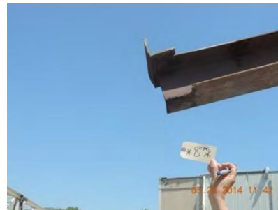
Fig. 33 – Joint 8 – South truss
