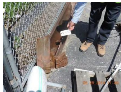
Fig. 39 – Joint 4 – East truss
