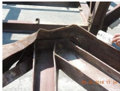
Fig. 21 – Joint 6 – North truss
