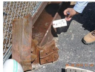
Fig. 29 – Joint 4 – South truss
