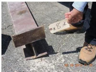
Fig. 23 – Joint 8 – North truss
