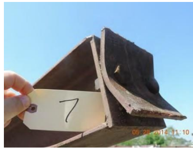
Fig. 71 – Joint 7 – South interior
