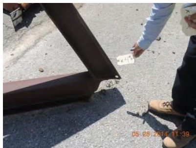
Fig. 28 – Joint 4 – South truss
