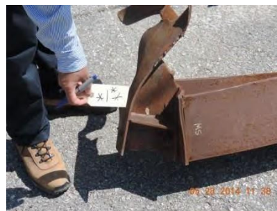
Fig. 24 – Joint 1 – South truss
