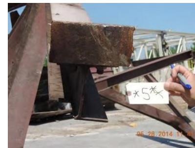
Fig. 30 – Joint 5 – South truss
