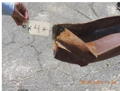
Fig. 19 – Joint 4 – North truss
