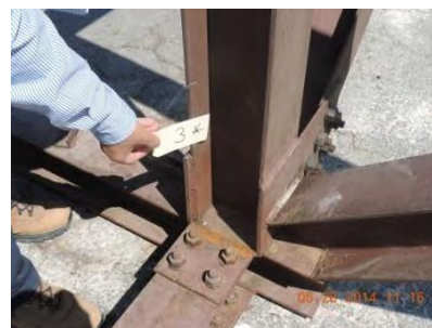
Fig. 54 – Joint 3 – East interior
