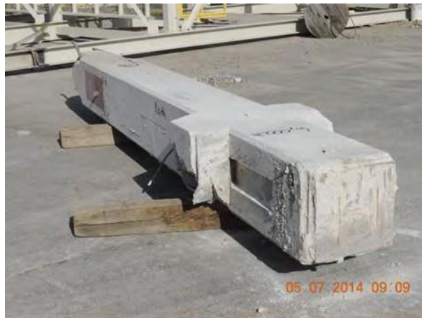
Fig. 95 – Intact column base plate
