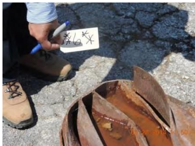
Fig. 41 – Joint 6 – East truss
