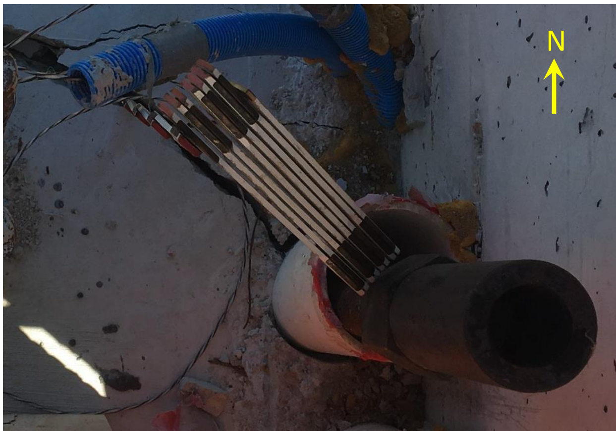
Figure 45 Note the gap indicative of movement between sleeve pipe and concrete, pictured on 3/13/2018 by BPA
