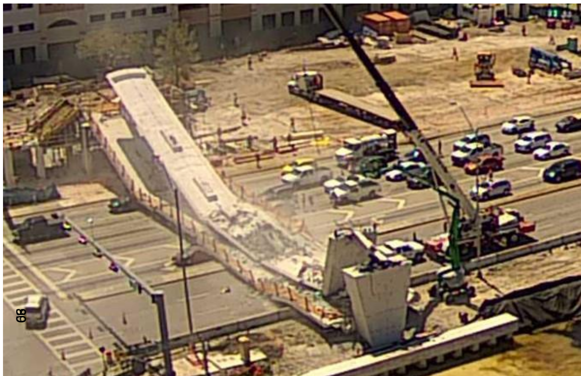
Figure 49 Bridge immediately after the collapse, March 15, 2018 – camera #2 Employees engaged in re-tensioning the PT bars in diagonal 11
