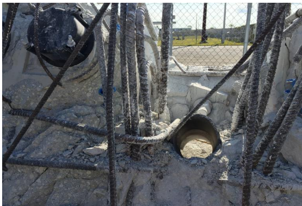
Figure 65 Punched hole in Diaphragm II at the time of the bridge collapse – from south looking towards
