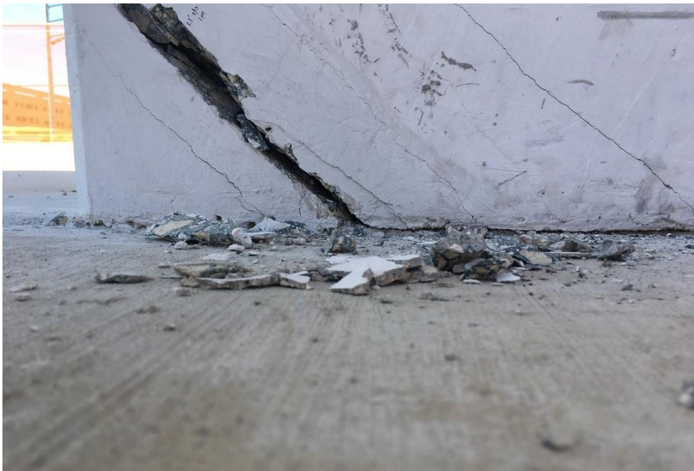
Figure 35 Cracks at the construction joint of the main span deck, diagonal 11 and the chamfer of diagonal 11 on 3/13/2018 by BPA
