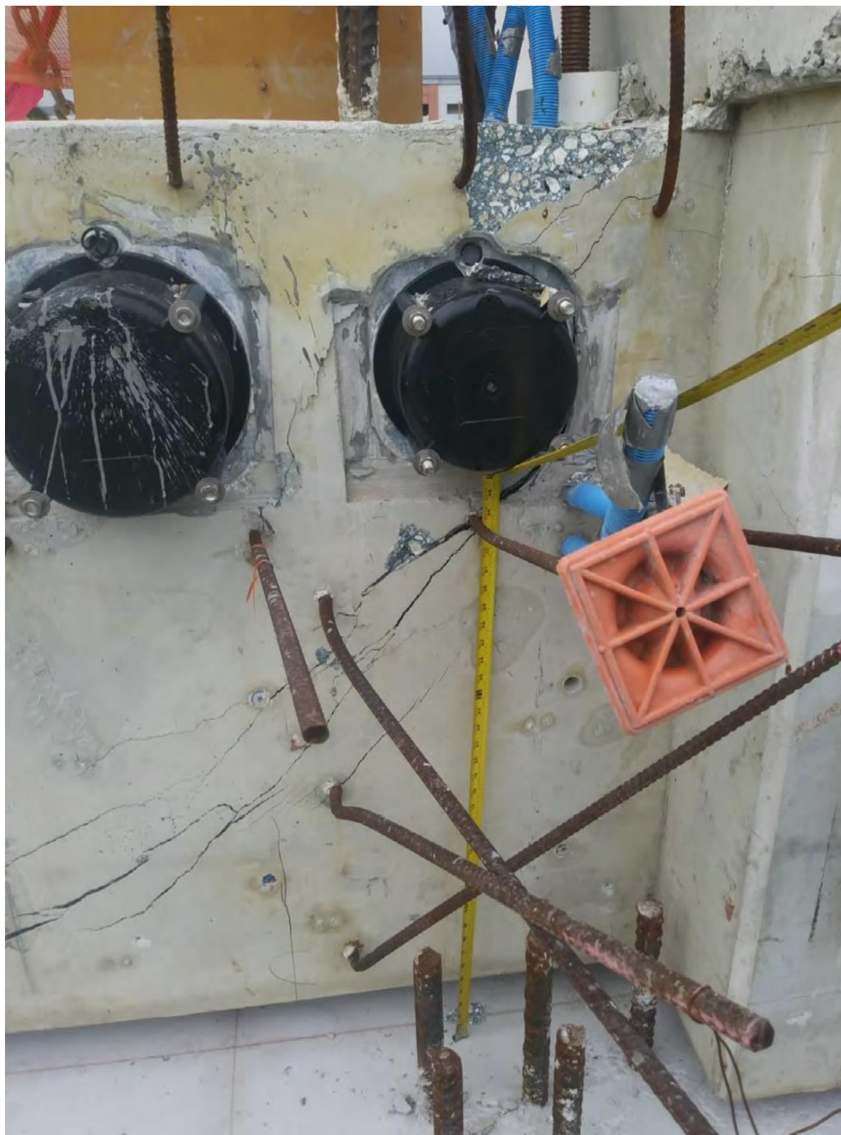
Figure 27 Cracks on the east side diaphragm II MCM email of 3/12/2018, by BPA – side face March 13, 2018 As the email was sent by MCM in the evening of March 12, 2018, FIGG did not open MCM's email containing the photos of the cracks until the next morning on FDA, Inc.
