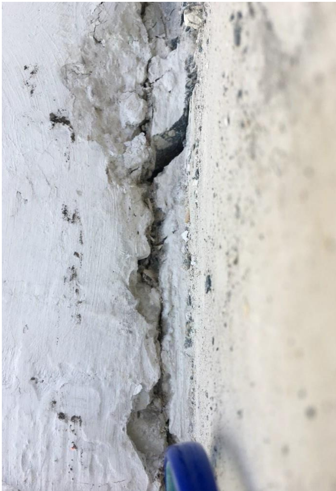
Figure 32 Cracks at the construction joint of the main span deck and diagonal 11 on 3/13/2018 by BPA
