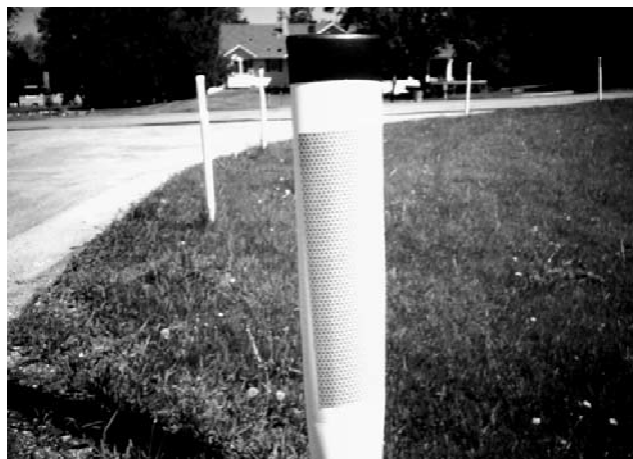
Culvert delineators are white with black at the top.
