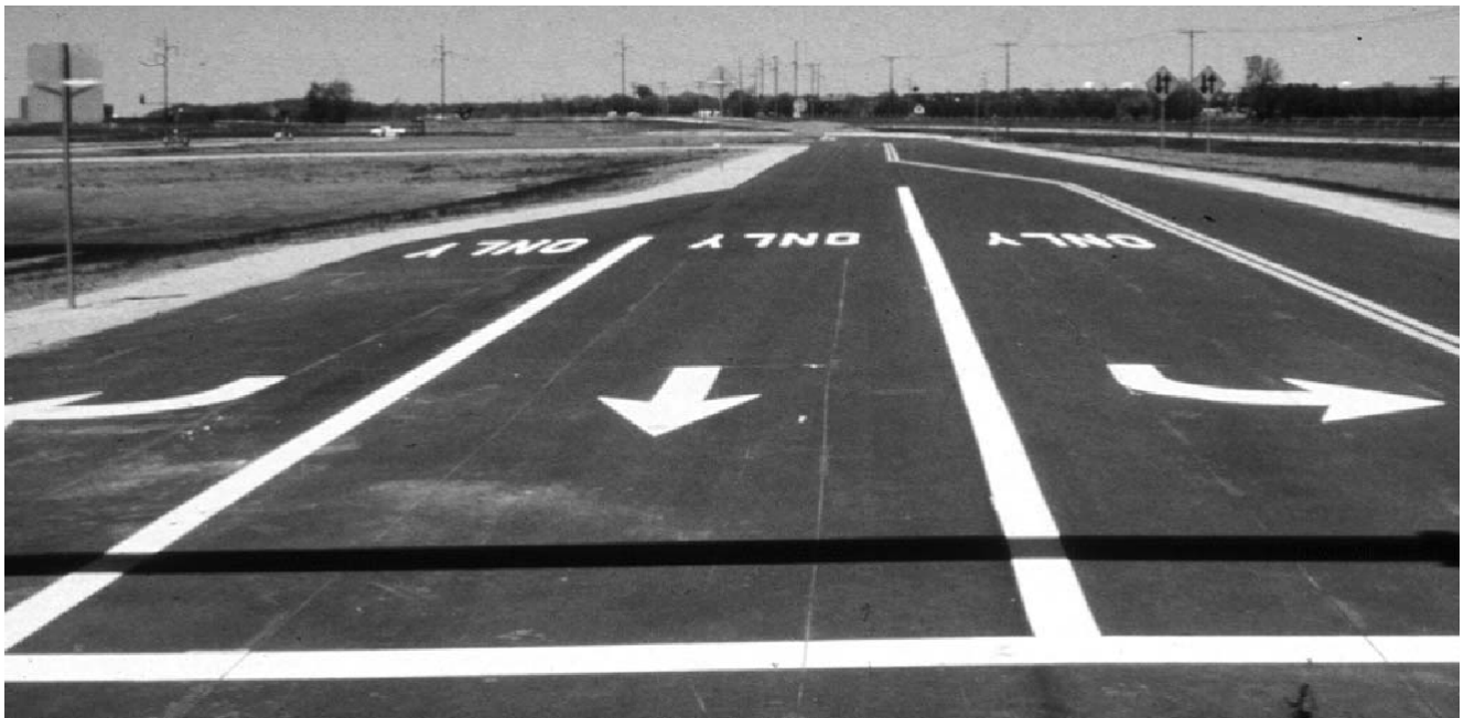
Arrow symbols channelize traffic at intersections where turns are mandatory.
