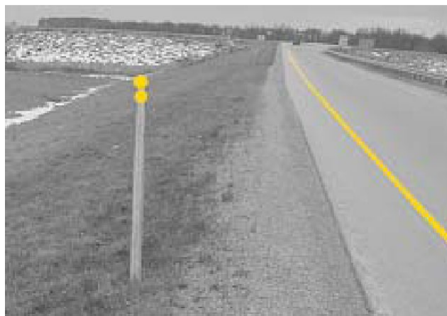
Delineators on the left side of a one-way road are yellow.
