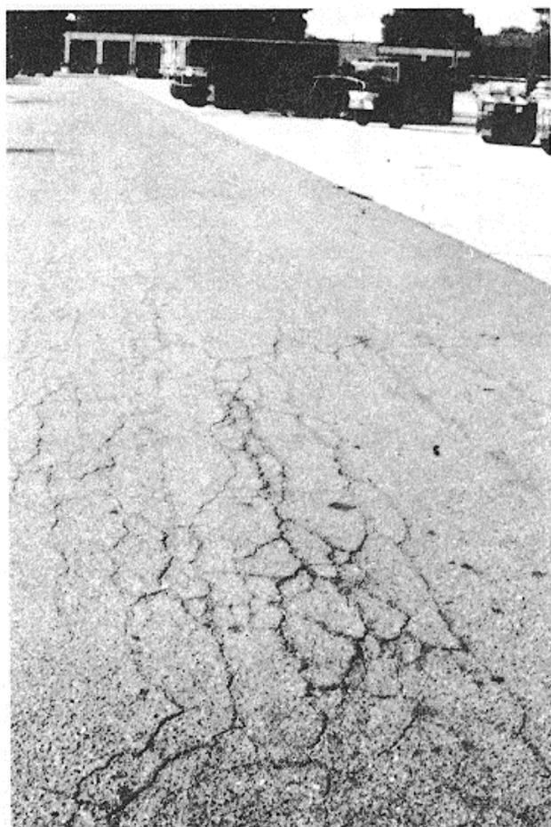
Figure B-3. Medium-severity alligator cracking
