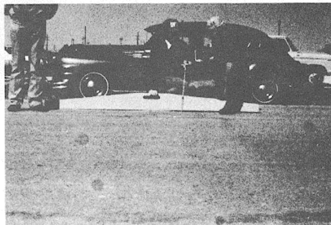
Figure B-24. Low-severity depression.
