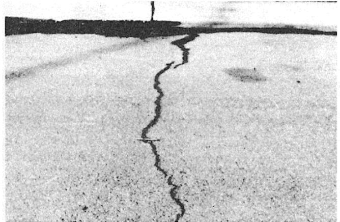
Figure B-39. Medium-severity longitudinal and transverse cracking.
