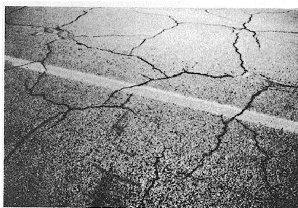
*Figure B-13. Medium-severity block cracking.*
