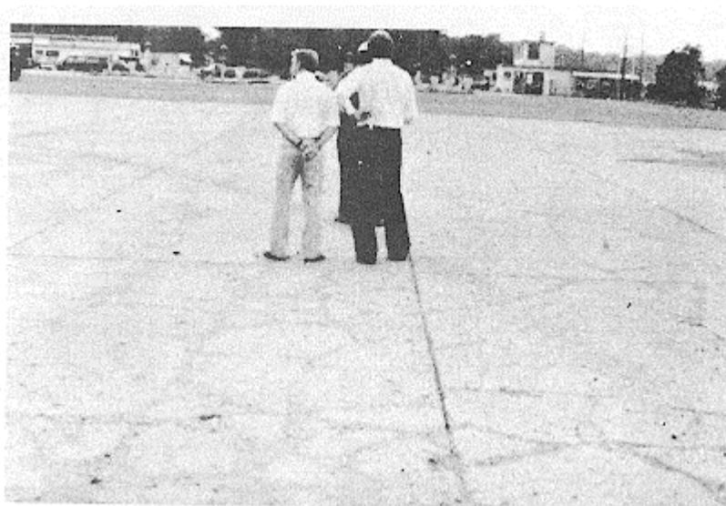
Figure B-84. High-severity divided slab.
