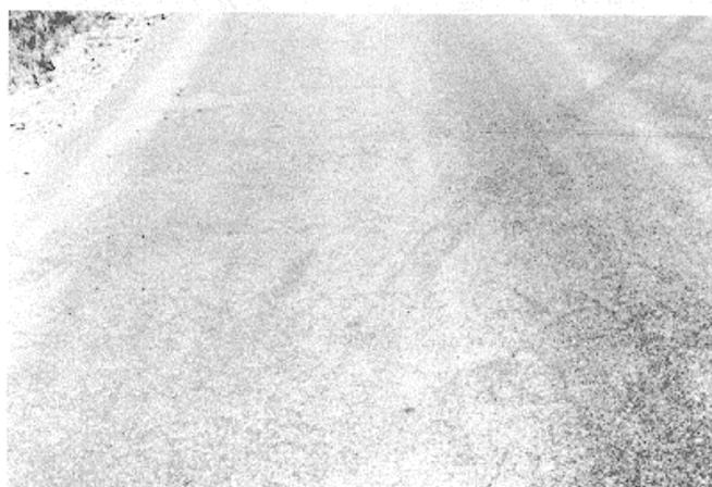
Figure B-8. Low-severity bleeding.
