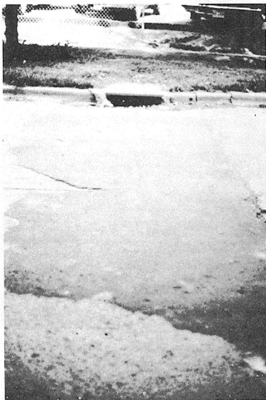
Figure B-110. Medium-severity patching, large.
