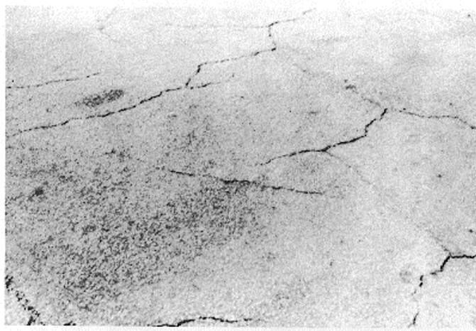
*Figure B-11. Low-severity block cracking.*
