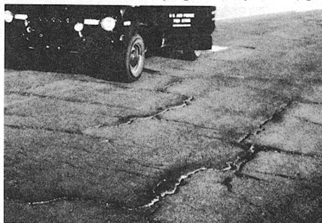
*Figure B-14. High-severity block cracking.*
