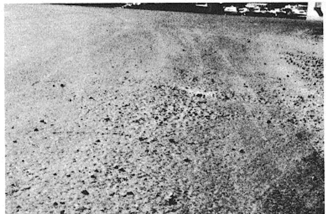
Figure B-70. Medium-severity weathering and raveling.
