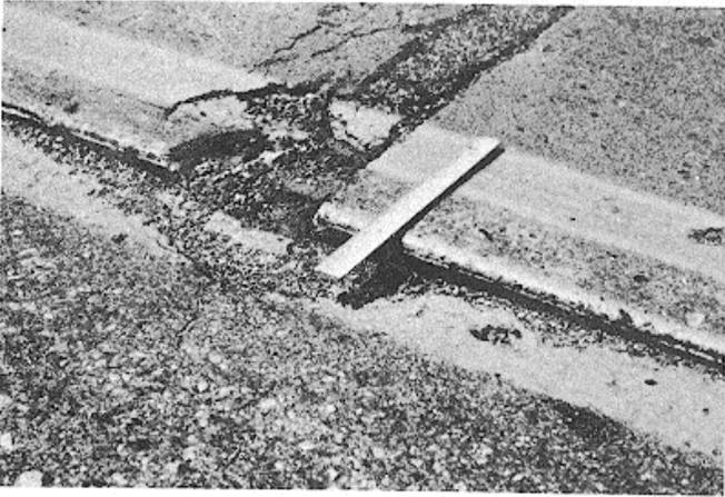
*Figure B-98. Low-severity lane/shoulder drop off.*
