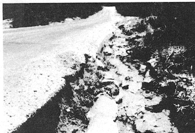
Figure B-37. High-severity lane/shoulder drop off
