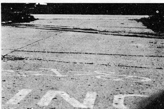
Figure B-124. Medium-severity railroad crossings.
