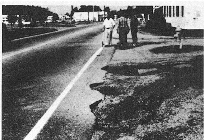
Figure B-29. High-severity edge cracking.
