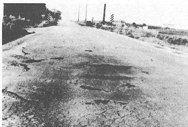
Figure B-61. Medium-severity shoving approaching high severity.
