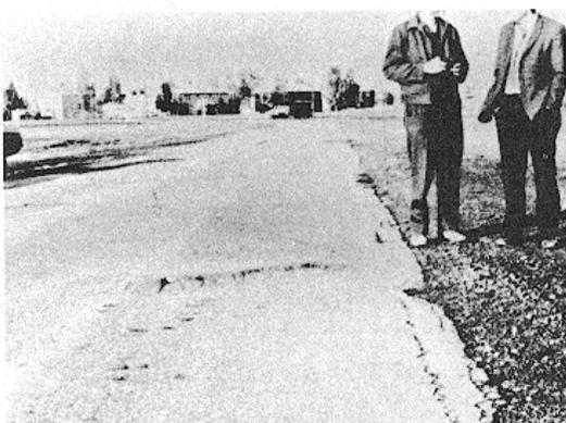
Figure B-16. Medium-severity bumps and sags.
