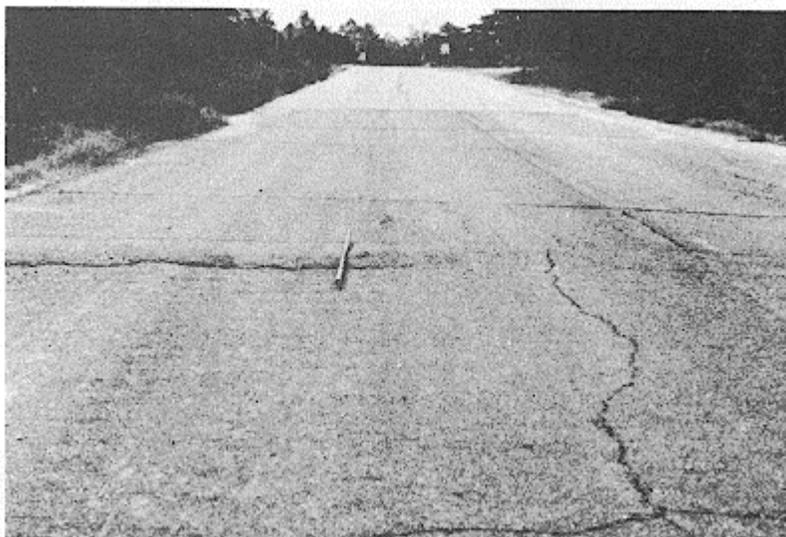
Figure B-18. Medium-severity bumps and sags.
