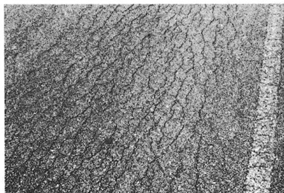
Figure B-5. Medium-severity alligator cracking.
