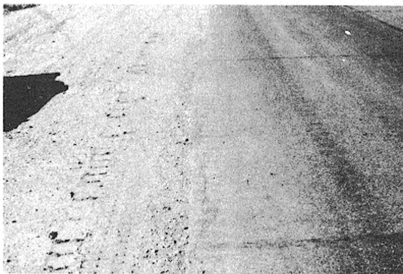
Figure B-31. Low-severity joint reflection cracking.
