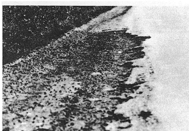
Figure B-30. High-severity edge cracking.
