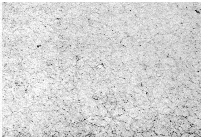
*Figure B-126. Low-severity scaling/map cracking/crazing.*
