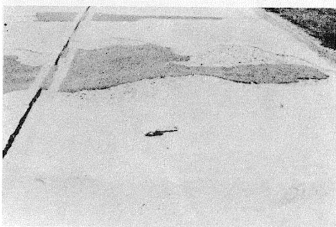
Figure B-128. High-severity scaling/map cracking/crazing.
