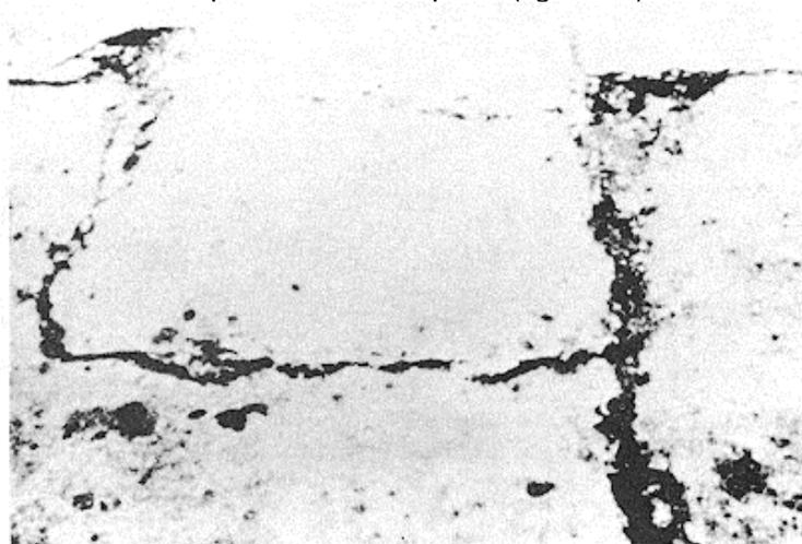
Figure B-112. High-severity patching, large.
