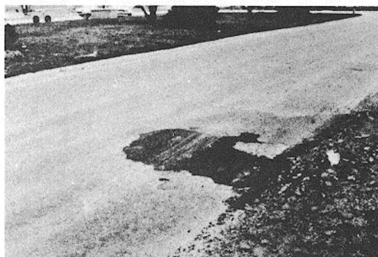
Figure B-45. Medium-severity patch.
