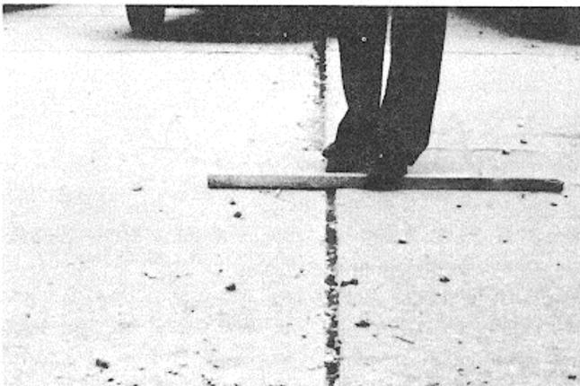
Figure B-90. Low-severity faulting.
