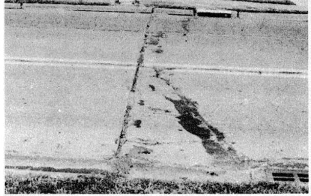
Figure B-121. Medium-severity punchout.
