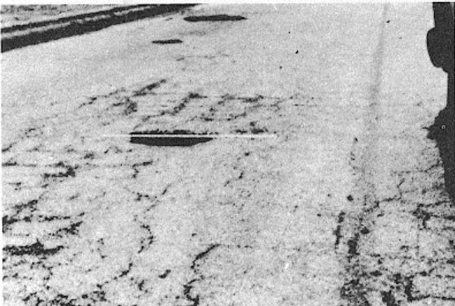
Figure B-50. Medium-severity pothole.
