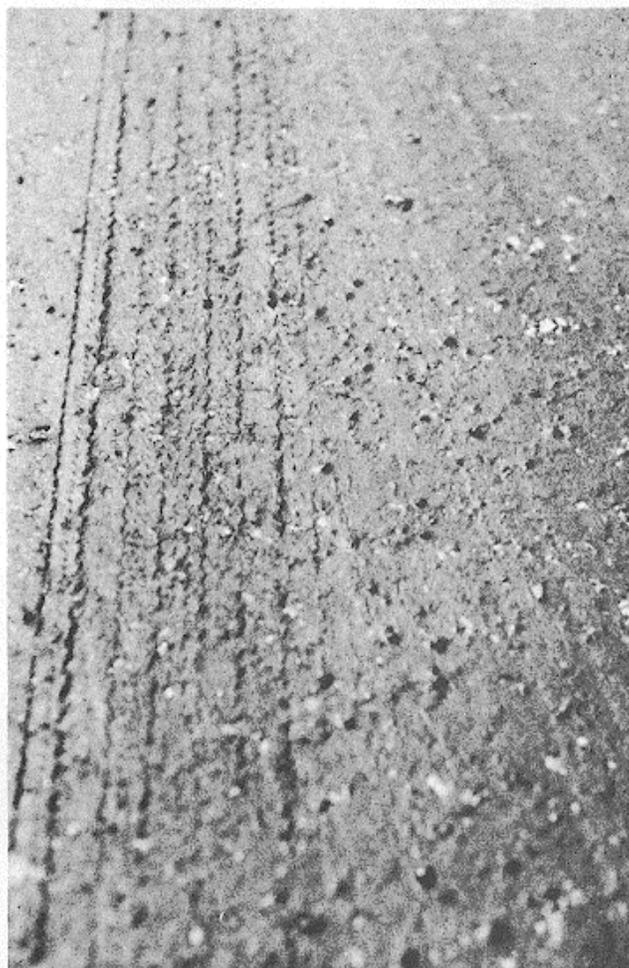
*Figure B-10. High-severity bleeding.*
