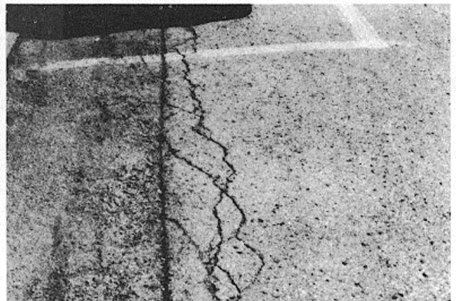
Figure B-28. Medium-severity edge cracking.
