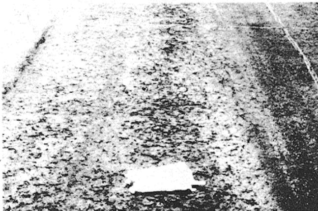
Figure B-69. Medium-severity weathering and raveling.
