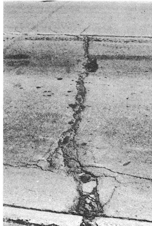
Figure B-41. High-severity longitudinal and transverse cracking.
