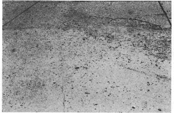
Figure B-89. High-severity durability cracking.
