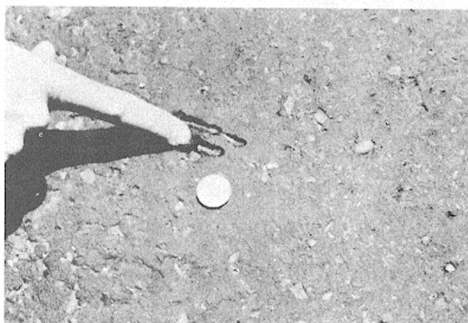
Figure B-9. Medium-severity bleeding.
