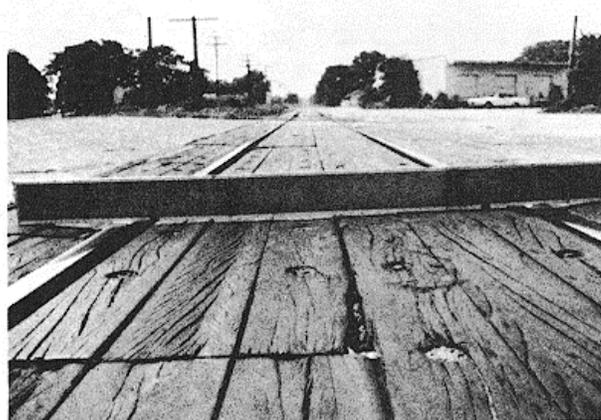
Figure B-53. Low-severity railroad crossing.
