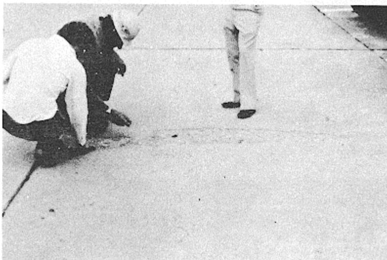
Figure B-87. Medium-severity durability cracking.
