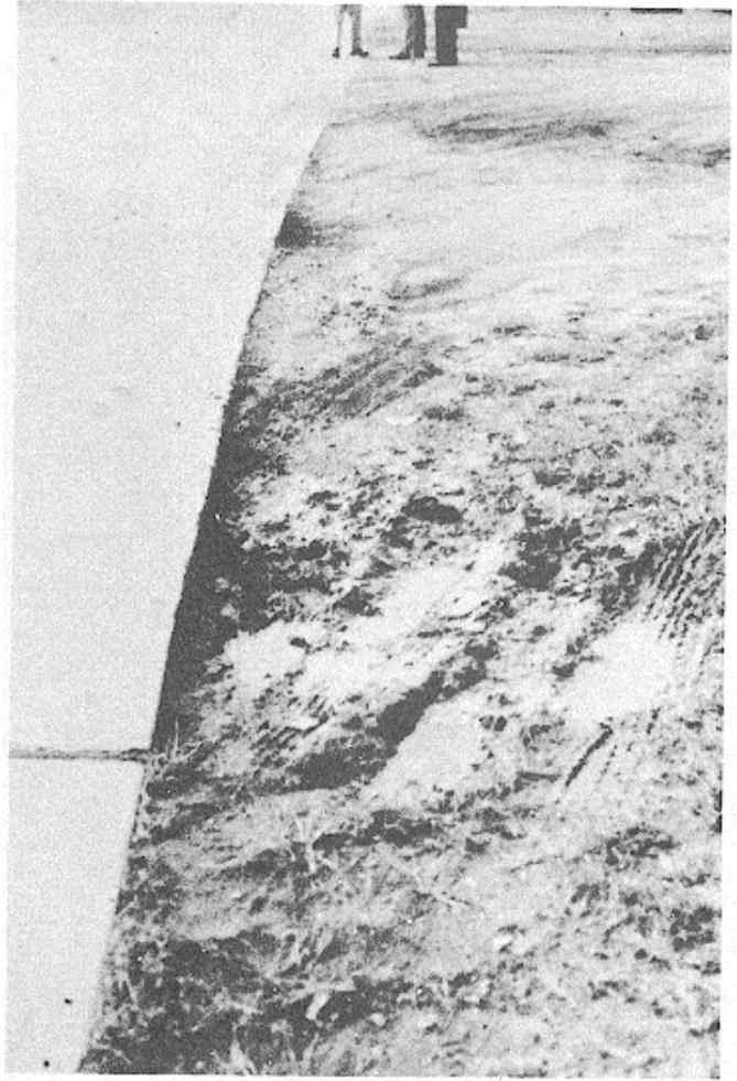
*Figure B-99. Medium-severity lane/shoulder drop off*
