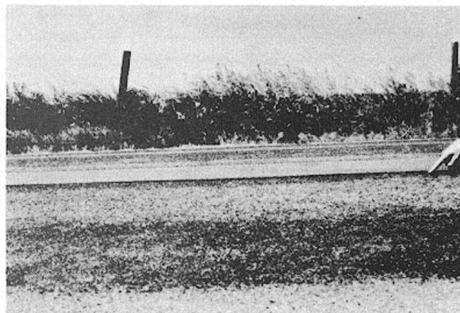
Figure B-20. Low-severity corrugation.
