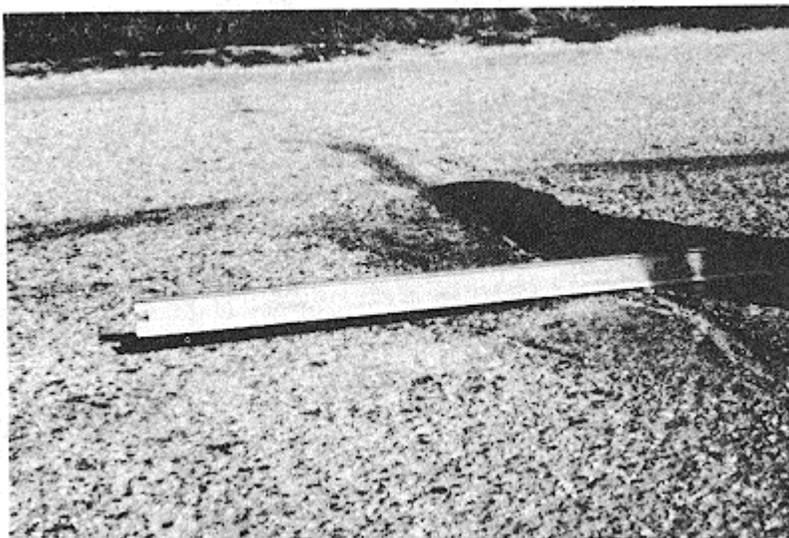
Figure B-15. Low-severity bumps and sags.
