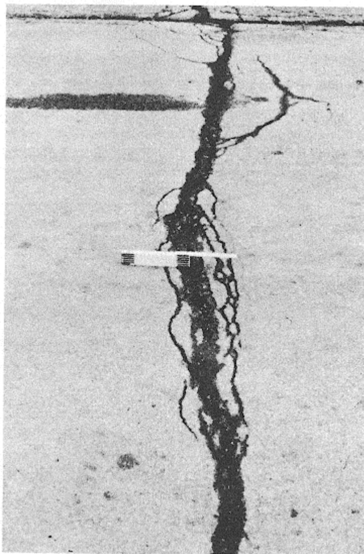
Figure B-33. High-severity joint reflection cracking.
