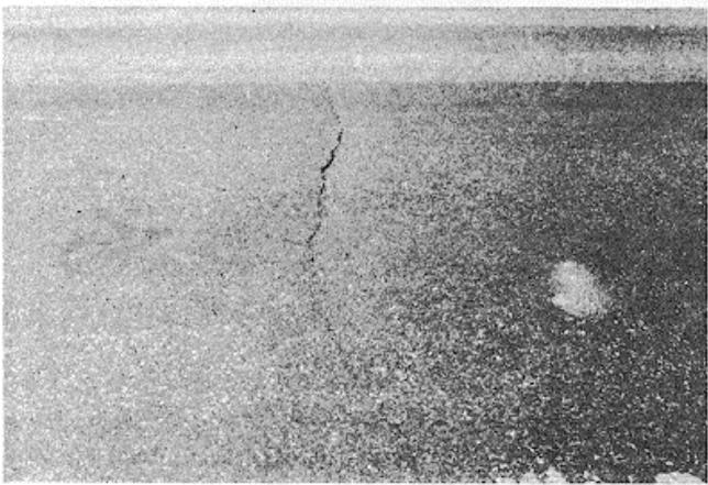
Figure B-38. Low-severity longitudinal and transverse cracking.
