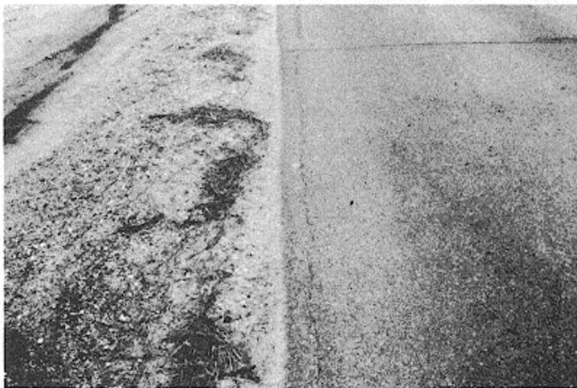
Figure B-27. Low-severity edge cracking.
