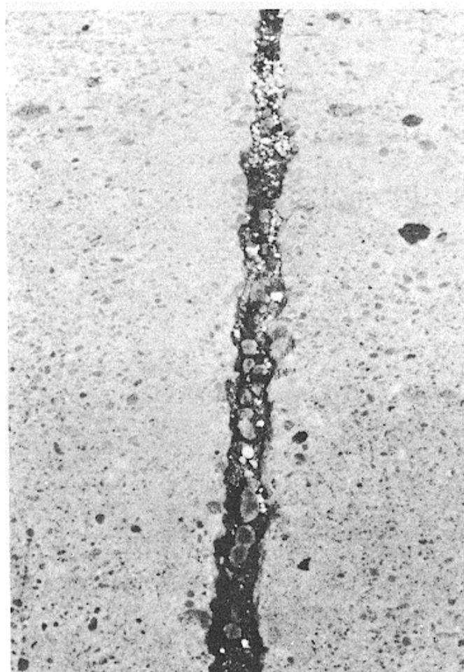
Figure B-97. High-severity joint seal damage.
