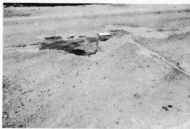
Figure B-129. High-severity scaling/map cracking/crazing.
