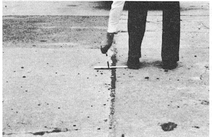
Figure B-91. Medium-severity faulting.
