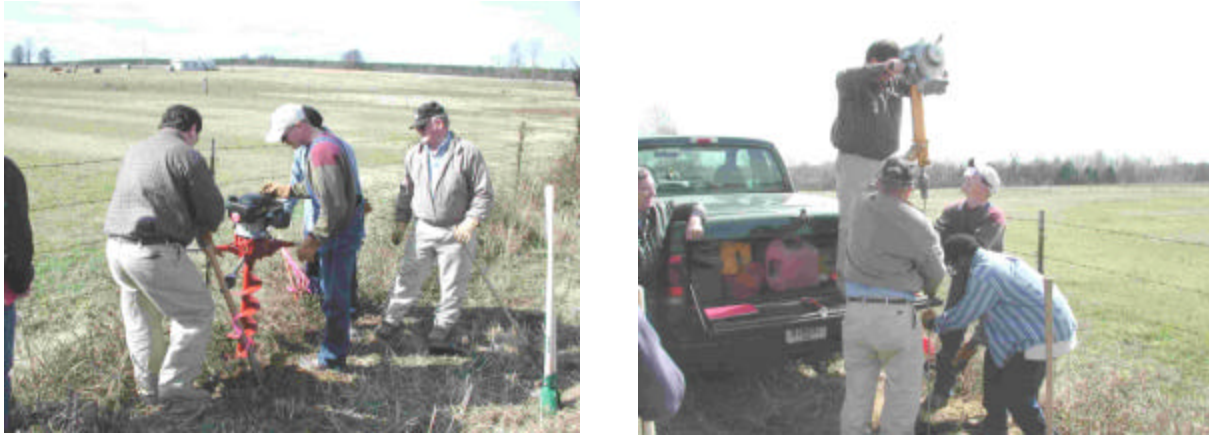
Figure 8-10. Setting deep-driven benchmarks (Memphis District & 3001, Inc.)
