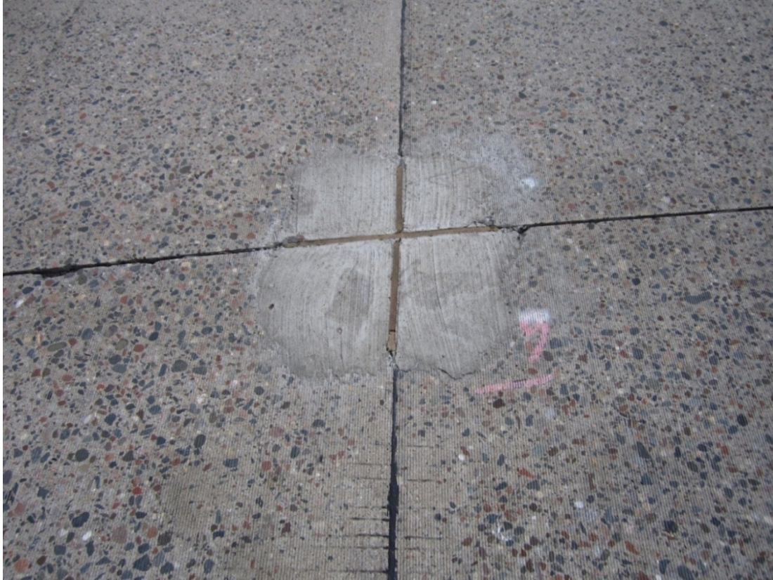
Figure 1.4. Typical MnROAD partial-depth repair with cementitious-based material.
