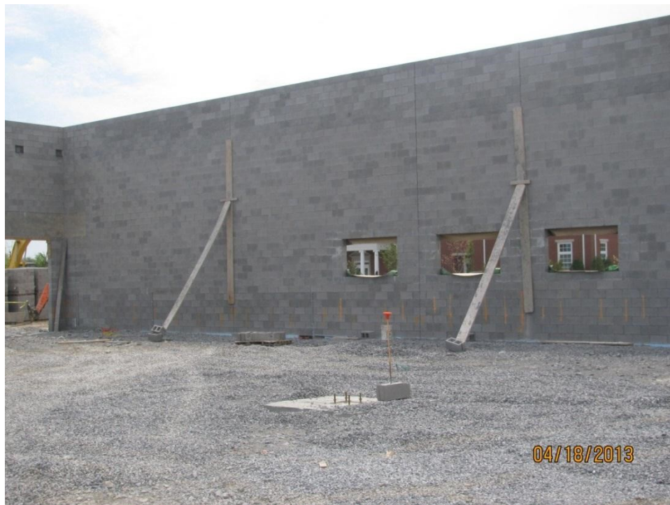
Figure 9 - Top end of brace without positive connection
