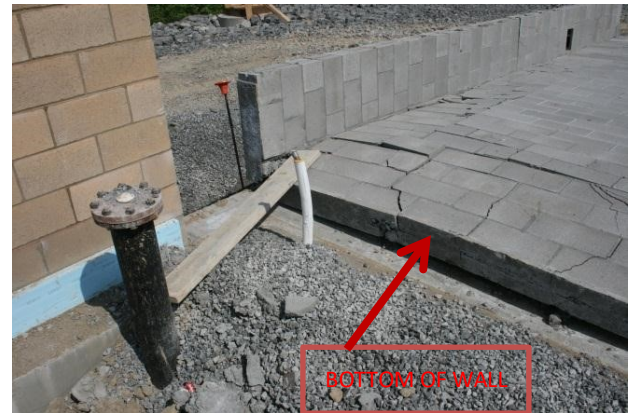
Figure 21 - Collapsed wall
