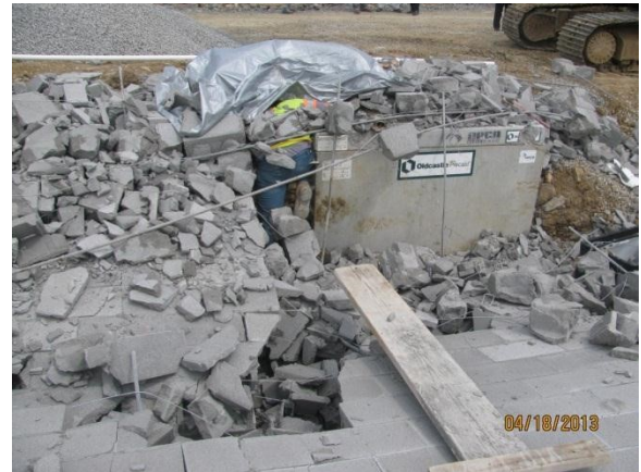
Figure 17 - Collapsed wall
