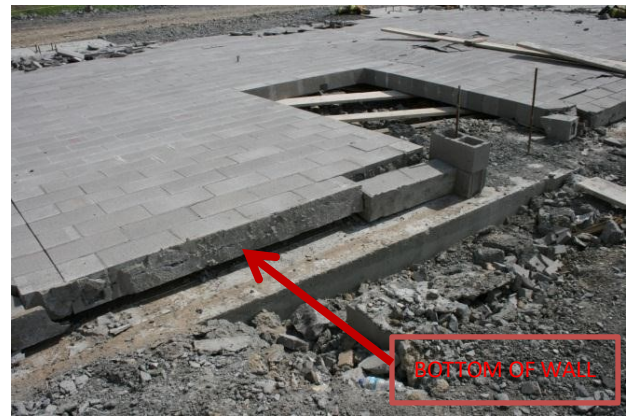
Figure 19 - Collapsed wall
