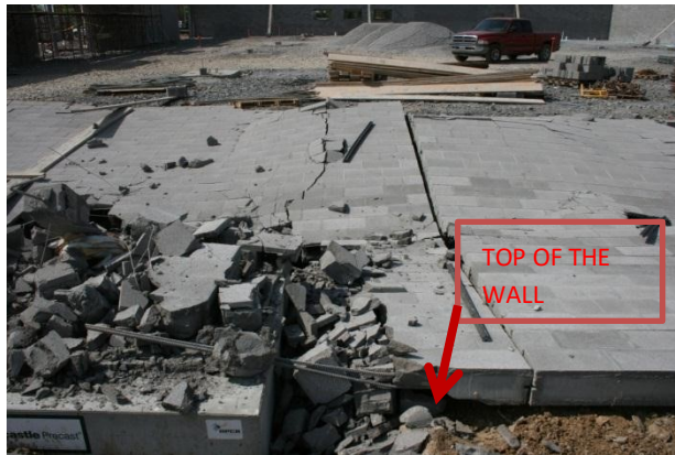
Figure 20 - Collapsed wall Structural Analysis and Discussion
