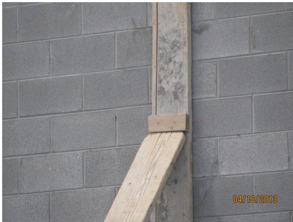
Figure 9 - Top end of brace without positive connection
