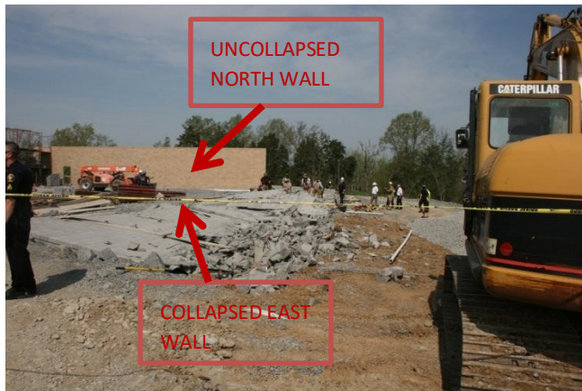
Figure 16 - Collapsed wall
