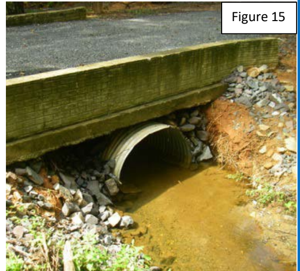
Figure 15: Inadequate culvert bedding combined with high flow depths causes piping; which is the loss of fill material. A headwall or riprap lining is needed.
