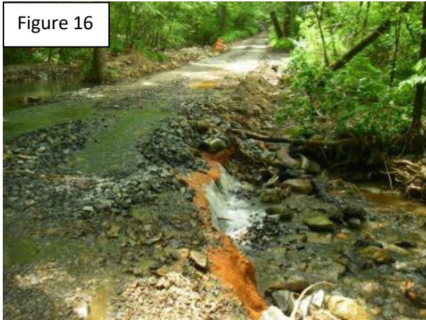
Figure 16: Frequent high flows that can clog and overtop the roadbed need a high water bypass; see practice specifications.
