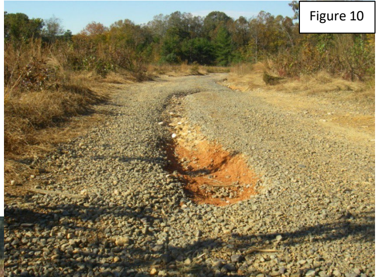
Figure 10: Erosion down the roadbed, see #1.
