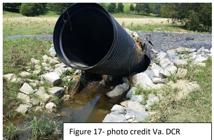
Figure 17: Poor placement of culvert resulted in buoyancy failure during high flow event. Culverts need 1 foot of cover and plastic pipes need to be weighted down.
