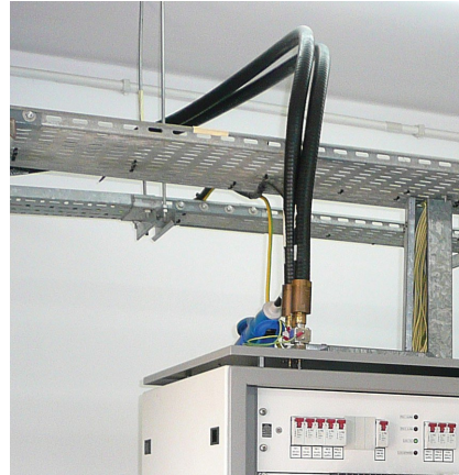
Figure 113. Incoming antenna circuits require protection.
