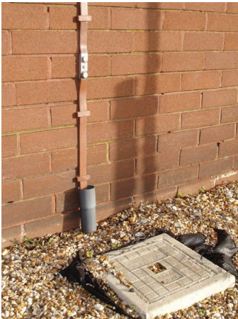
Figure 51. Typical down-conductor connectors.
