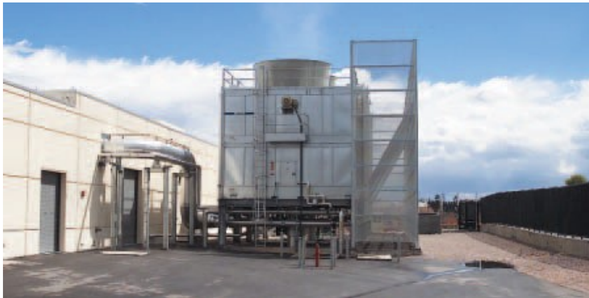
The LANL Nicholas C. Metropolis Modeling and Simulation Center currently uses treated wastewater from the LANL complex for cooling tower application.
