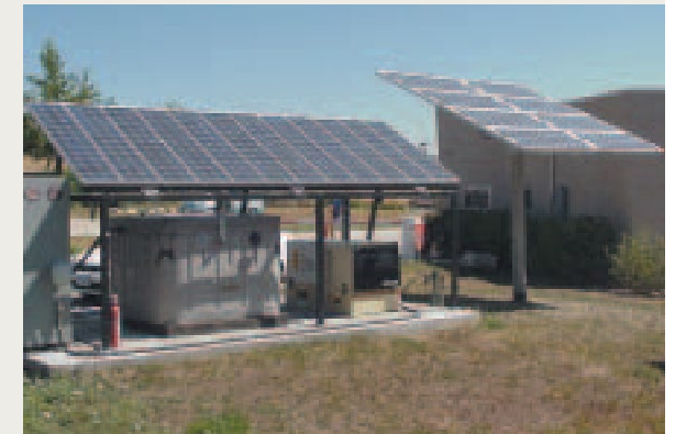
A PV/UPS system provides backup power for the Site Entrance Building at the National Renewable Energy Laboratory (NREL) in Golden, Colorado. The generator's 600-watt PV array charges a storage system of eight rechargeable batteries and enables NREL's security staff to maintain critical functions during power failures.
