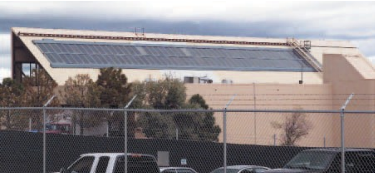
Solar hot water system on the LANL Otowi Building. The excellent solar resources in Los Alamos make solar hot water systems a viable solution for meeting DHW loads and preheating water for process and space heating loads. These systems have a high first cost, but very low operating costs. A year-round water heating load, such as for cafeteria, locker room facilities, and process loads, is required to make solar hot water systems cost-effective.
