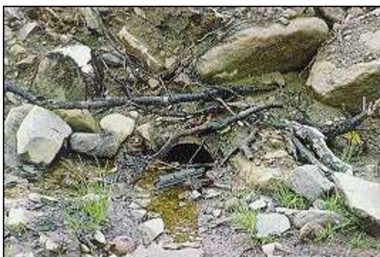
Undersized culverts can become plugged with sediment
