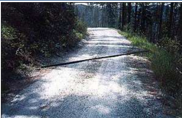
A deflector is an alternative method to divert surface water from a road.
