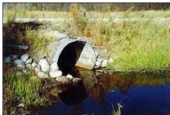
Culverts not installed at the same level as the stream cause water to back up.
