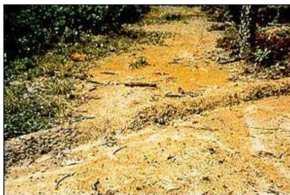
A water bar effectively intercepts surface water and diverts it from the road.
