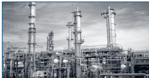
Fluid Heating in a Petroleum Process Heater
