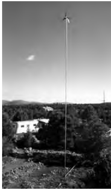
A Southwest Windpower Air 303, 300-watt turbine is the sole source of electricity for this remote home in northern Arizona.
