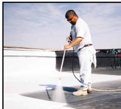
Figure 6: Two Cool Roof Installations
