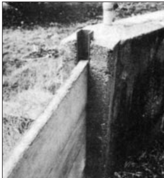
Figure 7-16 Slide-in closure panel.
