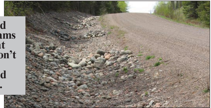
Figure 20: Rock check dam
