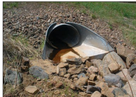
Figure 9: Most efficient, apron outlet
