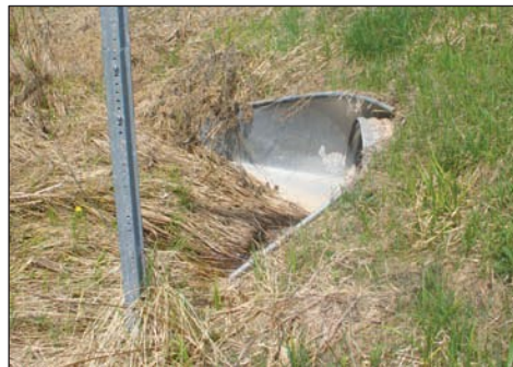
Figure 8: Most efficient, apron inlet
