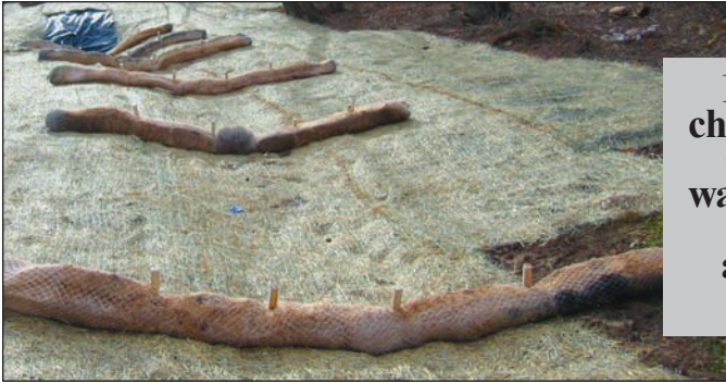
Figure 19: Bioroll check dam
