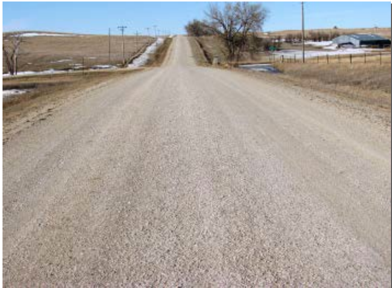
Example of very good surface gravel that has performed very well through the winter in the northern high plains.
