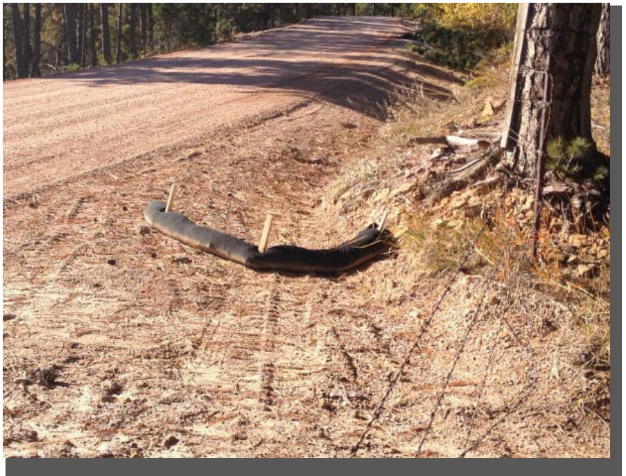
Good example of basic erosion control after gravel road reshape.
