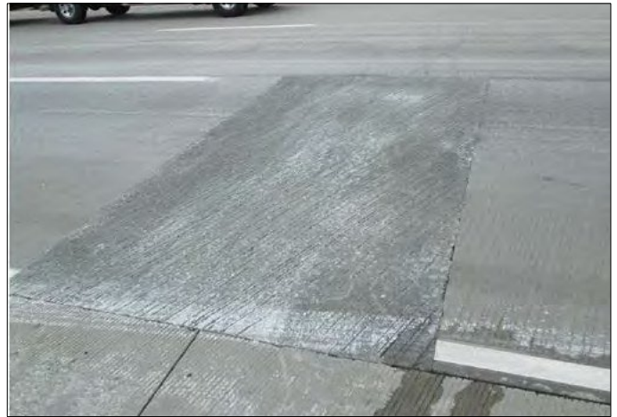
Figure 72. Completed FDR in CRCP.
