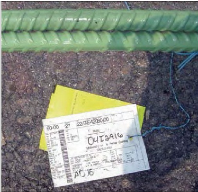
Figure 21. Mill and coating certifications for reinforcing steel.
