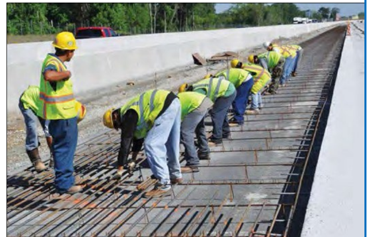
Figure 35. Placing longitudinal steel on TBAs.
