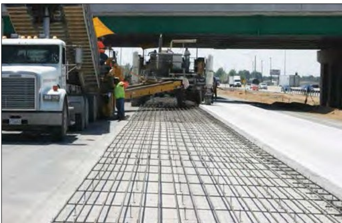
Figure 77. Unbonded CRCP overlay under construction.
