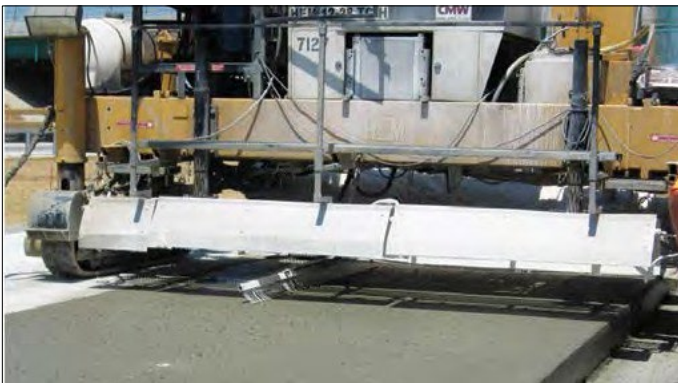
Figure 39. Applying transverse tining on a new CRCP.
