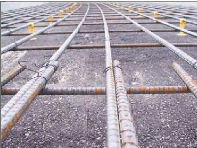
Figure 24. Lap splices.
