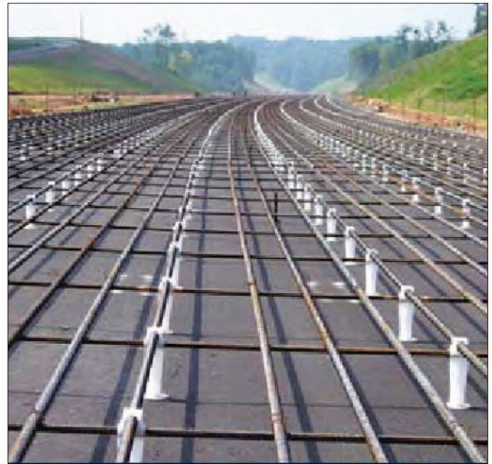
Figure 22. Steel placed on ATB (Virginia).
