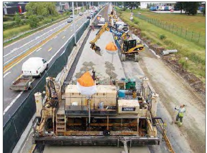
Figure 64. Construction of two-lift CRCP using two slip-form pavers on the A13 roadway (Belgium).
