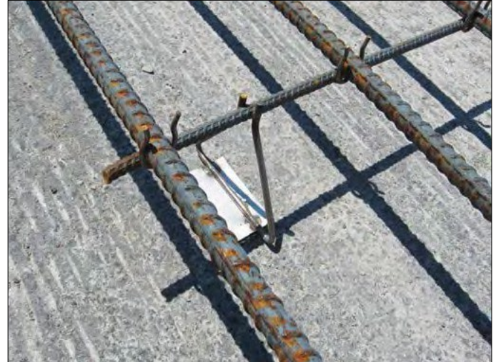
Figure 34. Transverse bar assembly (TBA).
