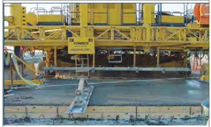
Figure 45. Finishing concrete at end-of-day header.
