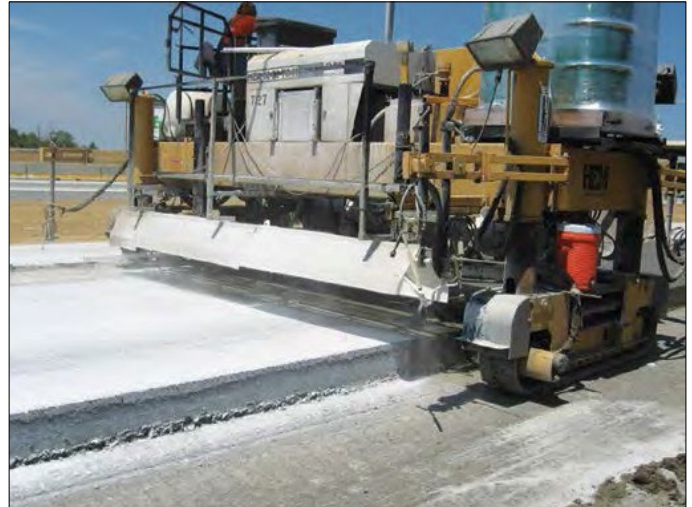
Figure 38. Application of curing compound on slip-formed CRCP.
