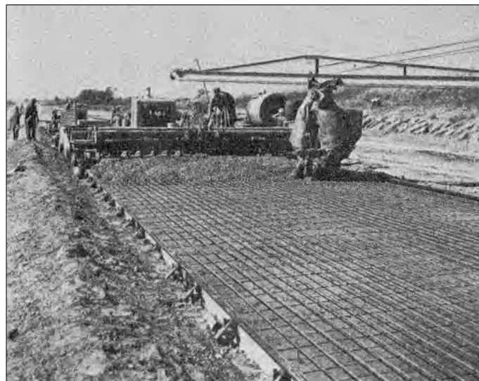
Figure 63. Construction of the 1947 Vandalia CRCP test sections (Illinois).
