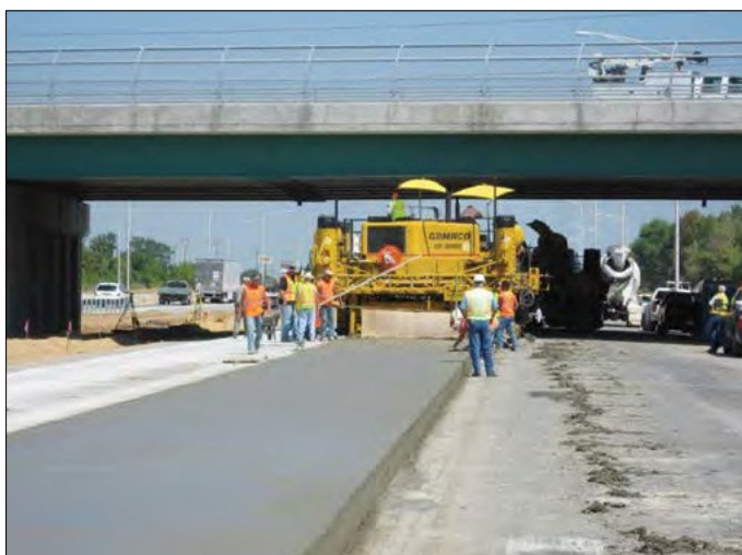
Figure 36. Slip-form paving of CRCP (Illinois).
