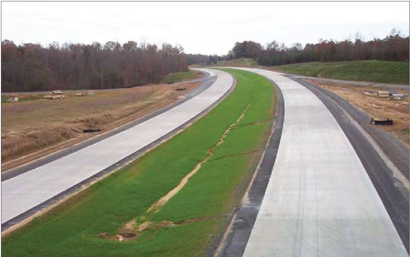
Figure 2. Newly constructed CRCP (Virginia).
