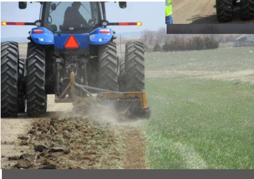
Example of a shouldering disk mounted on a tractor to process sod and gravel before moving it back to the road.
