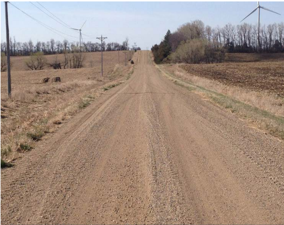
This is the same road as shown in the previous photo after complete surface and shoulder reshape and new surface gravel added. It performs well once again.
