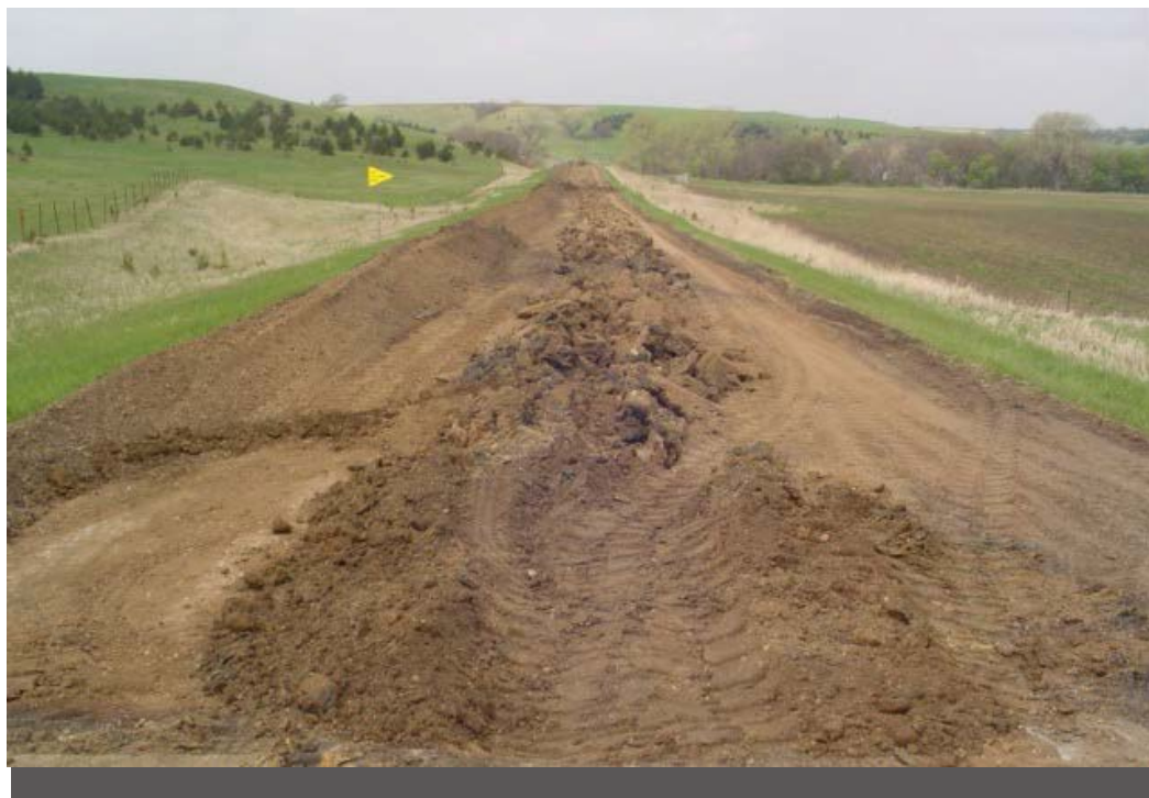
A road that had a constant problem with water percolating upward from springs beneath the surface. Work has just been completed to plow drainage pipe into the subgrade of this road.
