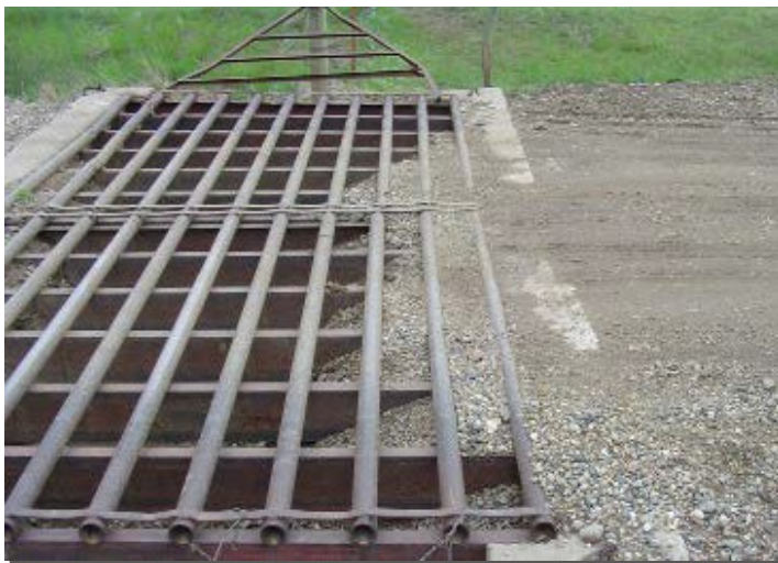
Care must be taken not to spill gravel into the cattle guard. Poor quality gravel with too much loose aggregate aggravates the problem of material spilling into the cavity.
