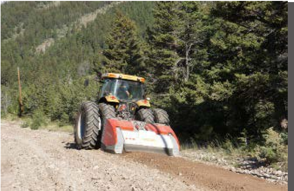
An example of a tractor-mounted crusher processing coarse material in-place.
