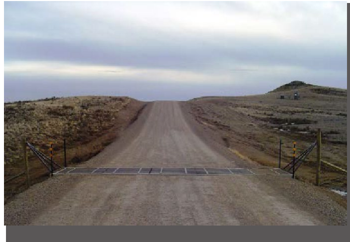
Road is shaped very well for a smooth crossing over the cattle guard.
