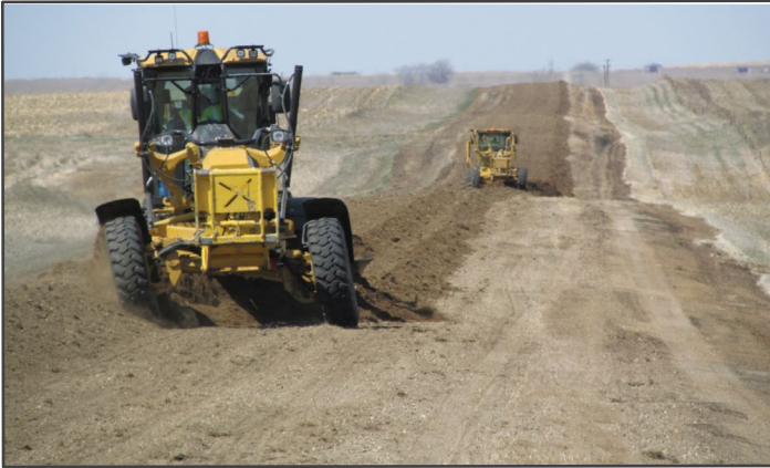
Reconstruction work space. (Source: Greg Vavra, SDLTAP).
