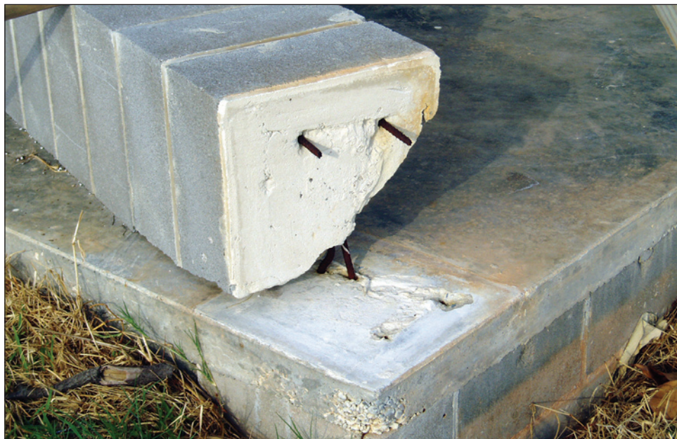
Figure 2-6. Column connection failure (Belle Fontaine Point, Jackson County, Mississippi)
