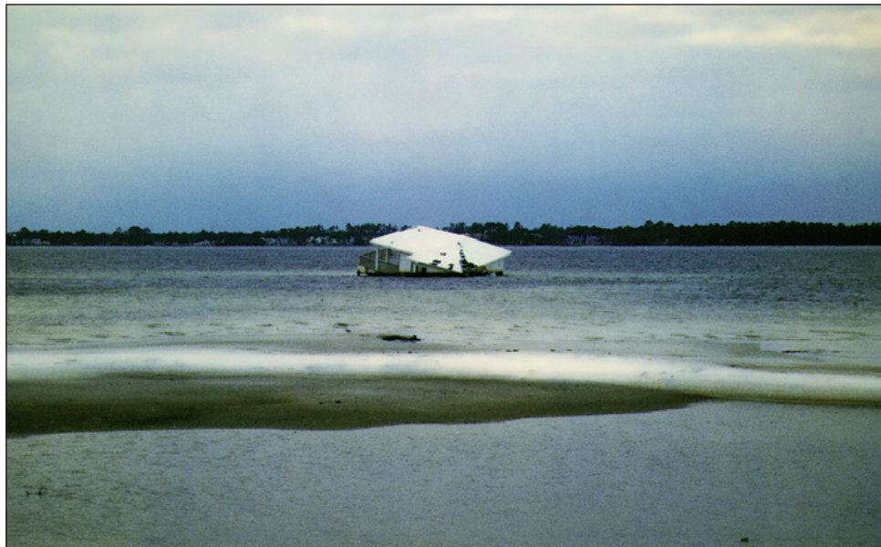
Figure 1-9. During Hurricane Opal (1995), this house was in an area of channeled flow between large buildings. As a result, the house was undermined and washed into the bay behind a barrier island.
