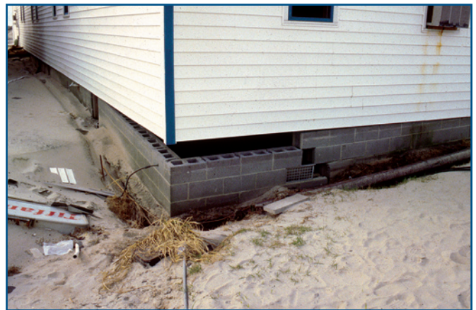
Failure of crawlspace foundation undermined by scour.
