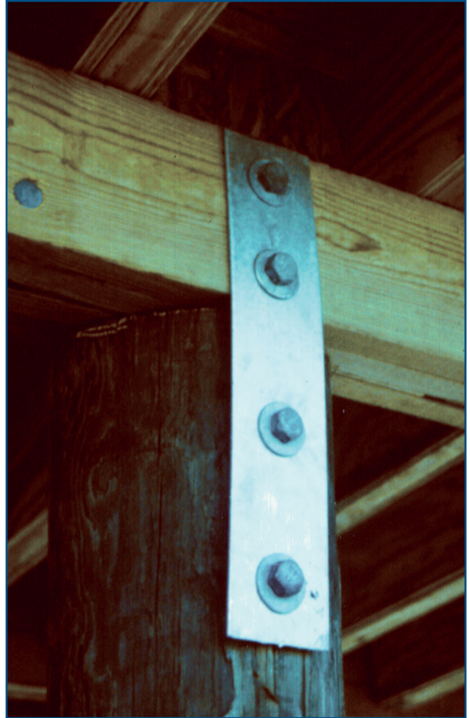
Metals corrode at a much faster rate near the ocean. Always use well-protected hardware, such as this connector with thick galvanizing. (For information about pile-to-beam connections, see Fact Sheet No. 13).
