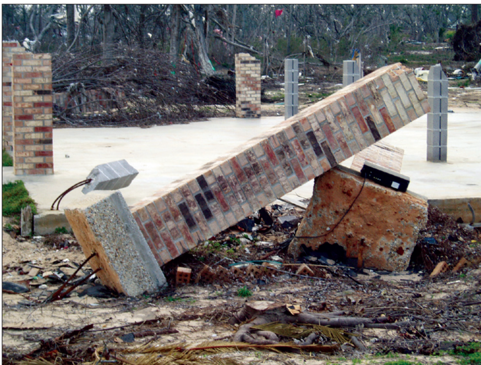
Figure 2-7. Performance comparison of pier foundations. Piers on discrete footings (foreground) failed by rotating and overturning while piers on more substantial footings (in this case a concrete mat) survived (Pass Christian, Mississippi)
