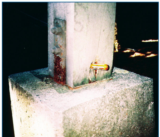
Metals corrode at a much faster rate near the ocean. Always use well-protected hardware, such as this connector with thick galvanizing. (For information about pile-to-beam connections, see Fact Sheet No. 13).
