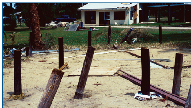
Insufficient pile embedment and failure of connections at tops of piles allowed elevated building to be floated off its foundation.
