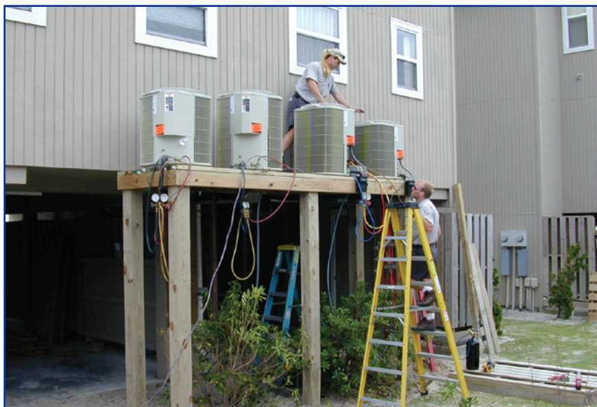
Elevated air conditioning compressors.
