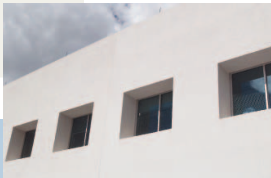
Placing the windows deep in the south-facing wall helps to shade the window to minimize direct solar gains and reduce perimeter cooling loads.
