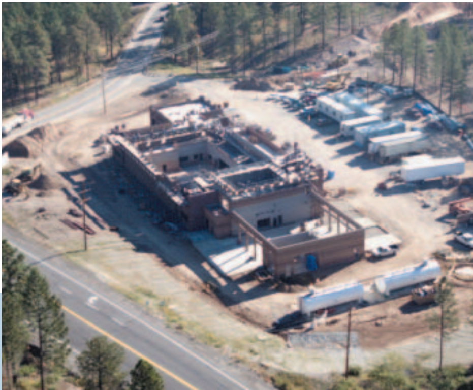
CMU construction for the LANL Emergency Operations Center provides a durable exterior wall. A second CMU interior wall provides mass to improve interior thermal comfort.
