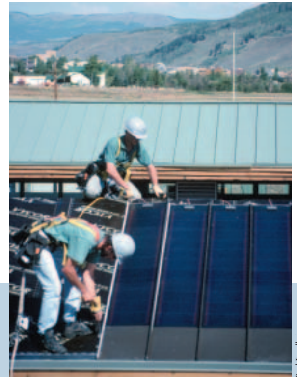
The method for installing a PV-integrated standing seam metal roof is the same for a similar type roof without PV.
