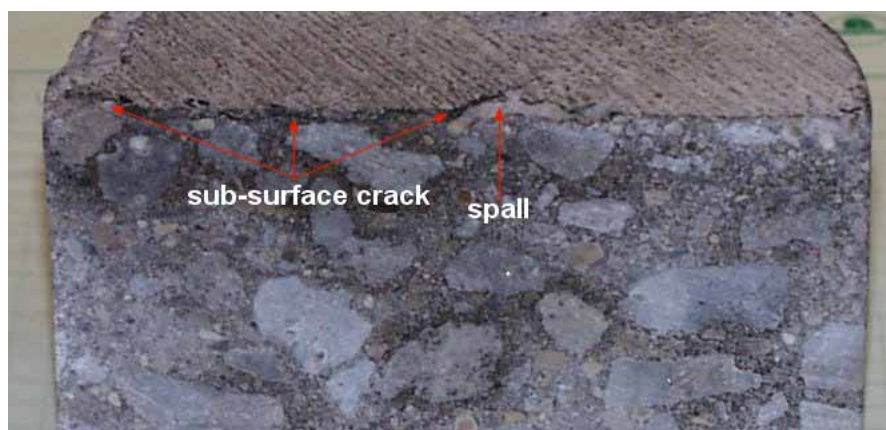
Figure 15. Development of spall as a result of early application of curing compound.
