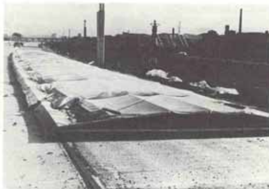
Figure 1. Canopy used to protect fresh concrete.
