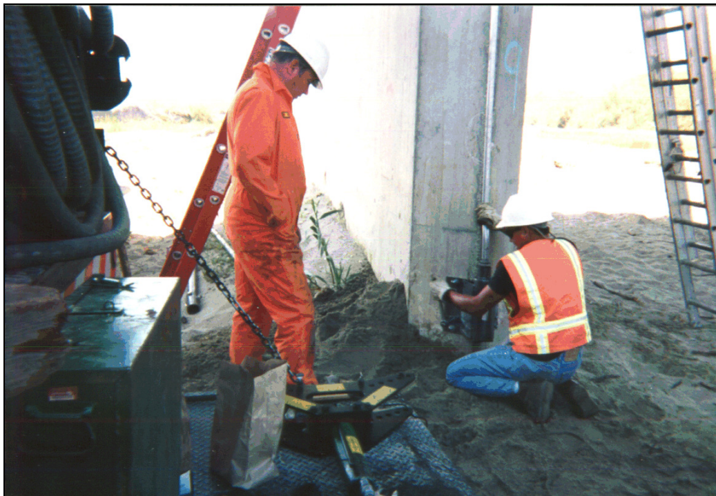
Figure 9.27. Installation of a sonar scour monitor on Salinas River Bridge near Soledad, California (Highway 101) by CALTRANS.
