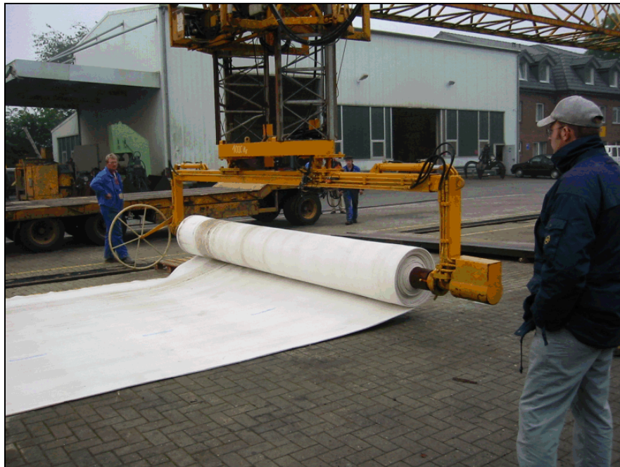
Figure 5.3. SandMat™ geocomposite blanket being unrolled. (photo from NCHRP Project 24-07(2), courtesy Colcrete – Von Essen Inc.)
