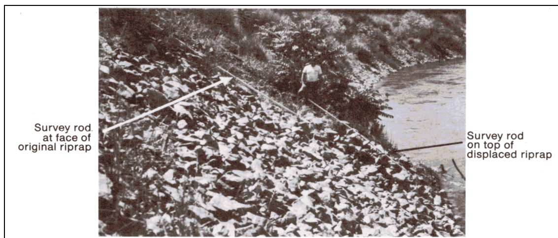
Figure 5.13. Riprap on Consumnes River at Site 3 near Sloughhouse, CA, looking downstream, showing modified slump failure (photographed May 31, 1983) (Blodgett & McConaughy 1986).
