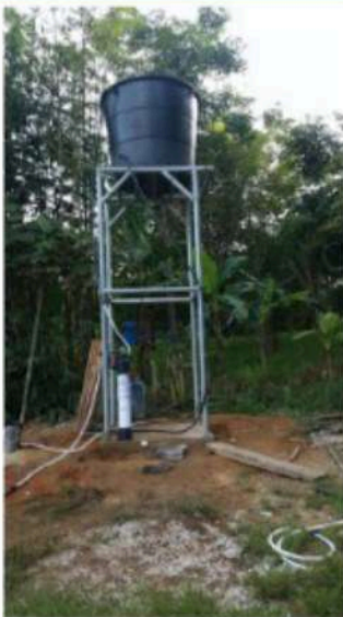
Fig. 1: Install water storage tanks with RFU*
