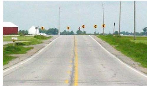
After installation of Chevrons.
