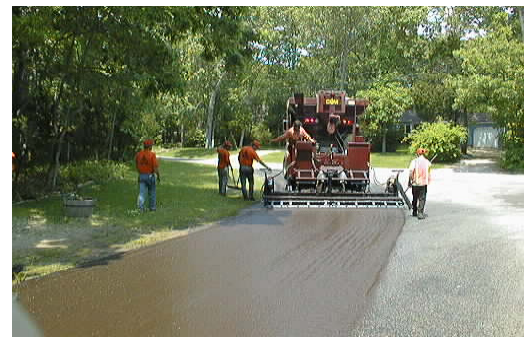
Application of skid-resistant pavement surface in curve.
