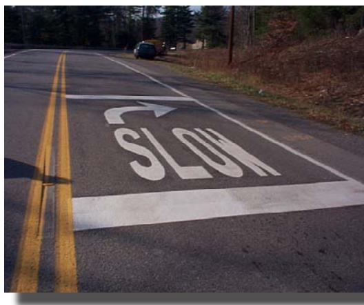
PennDOT curve advance marking.
