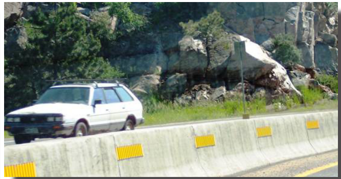
Reflective sheeting shaped to provide linear reflectorization.
