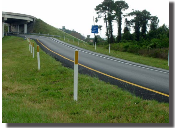
Post delineators installed on a ramp.
