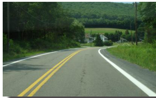
Roadway with 8-in edge line
