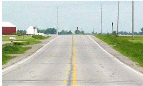
Before installation of Chevrons.
