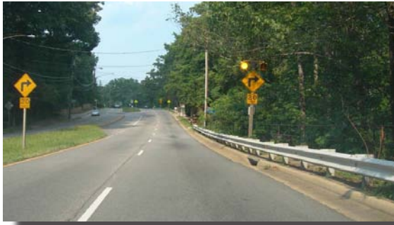
Doubling-up of the sign proved effective at this site because tree limbs partially blocked the right side sign.
