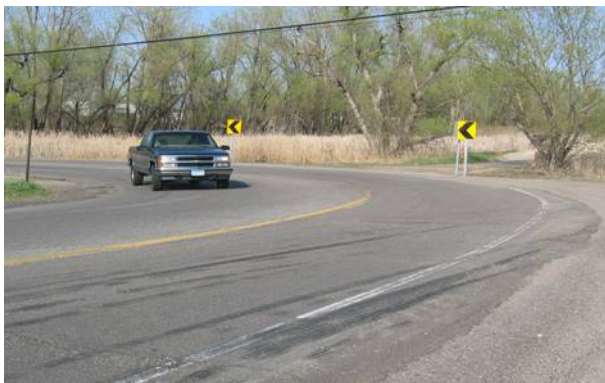
Widening on inside of curve.
