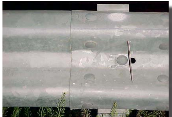
Installation of reflectors on W-beam guardrail.
