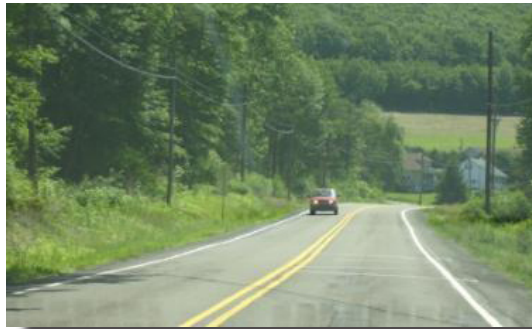
Roadway with 4-in edge line
