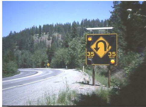
Flashing Beacon on Warning Sign.
