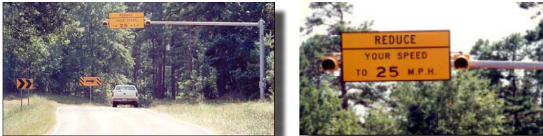
Dynamic curve speed warning system in Camp County, Texas.
