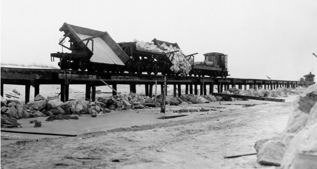
Figure I-3-6. Construction of Fire Island jetty on Democrat Point, at the west end of Fire Island, Long Island, New York. Many early USACE jetties were built from the land moving seaward using materials brought in by train. Photograph taken 3 Jan 1940, from Beach Erosion Board Archives.
