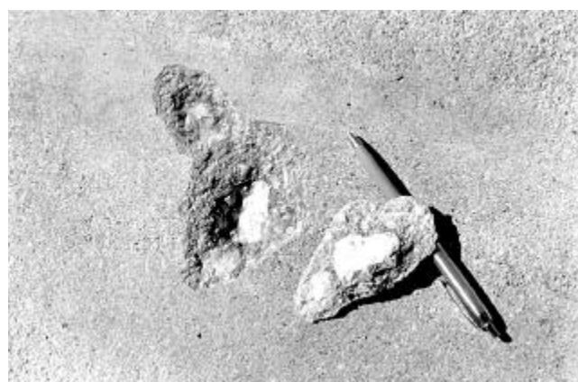
Fig. 11.6—A popout is a small fragment of concrete broken away from the surface of a slab due to internal pressure, leaving a shallow, typically conical, depression
