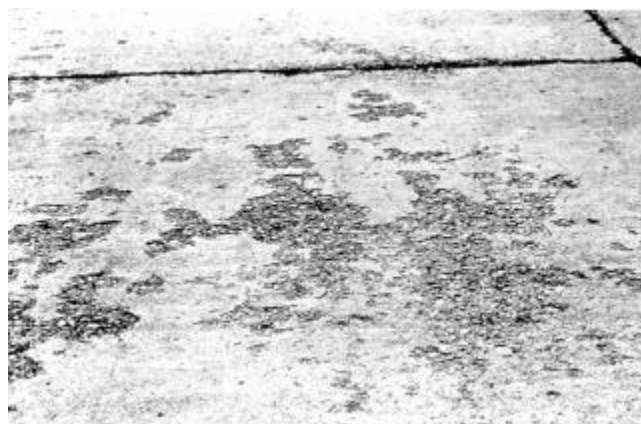
Fig. 11.5—Scaling is the loss of surface mortar, usually exposing the coarse aggregate
