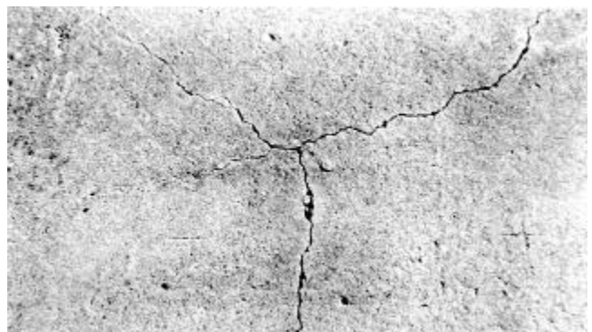
Fig. 11.2—Drying shrinkage cracks such as these are a frequent cause of complaint
