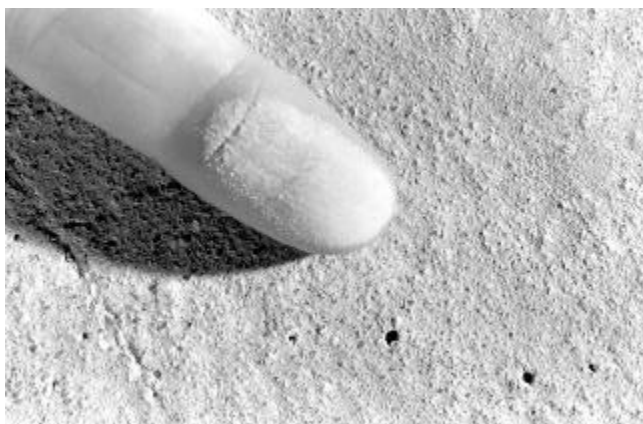
Fig. 11.4—Dusting is evident when a fine powdery material can be easily rubbed off the surface of a slab
