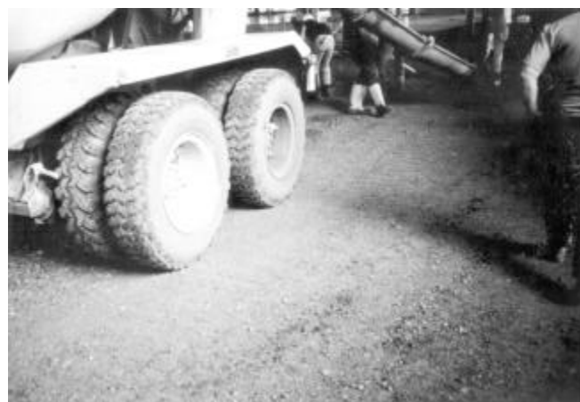
Fig. 4.1.1—Proofrolling by loaded ready mix truck
