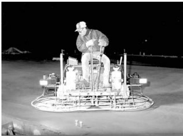
Fig. 8.2.4.4—Double-riding trowel with clip-on pans
