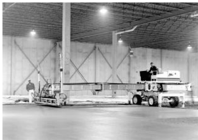
Fig. 8.2.3.2—Laser controlled screed
