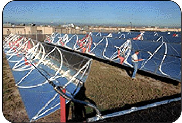
Solar water heating is a proven technology that directly substitutes renewable energy for conventional water heating. This array of parabolic trough collectors was paid for through an Energy Savings Performance Contract (ESPC).
