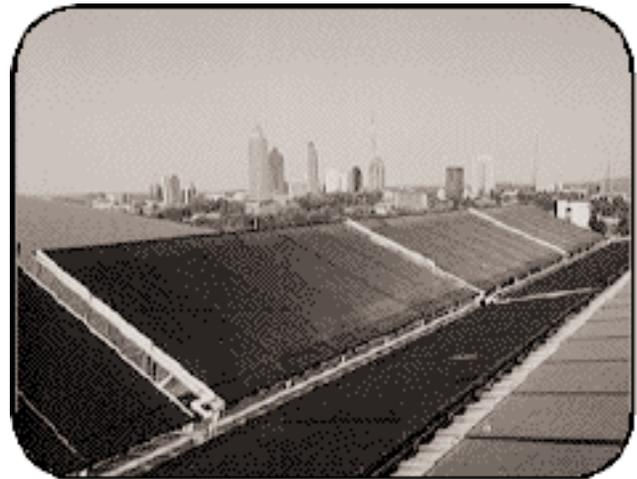
Solar thermal water heating can meet hot water demand at very low operating cost. Flat plate collectors are in the middle of the photo. Also shown are PV panels on the flat portion of the roof.
