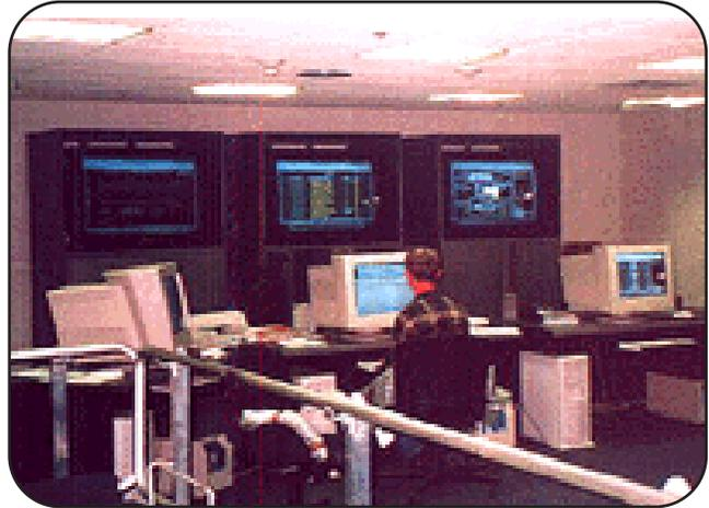
Energy Management and Control Systems can monitor and control equipment throughout a facility from a single location.
