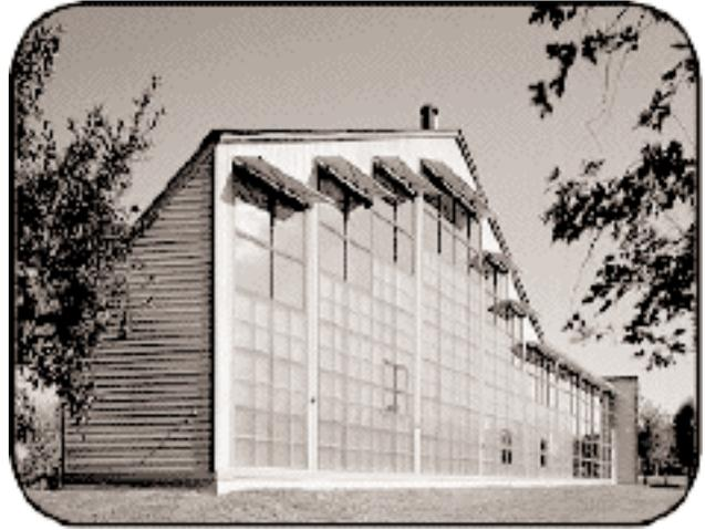
This passive solar building incorporates trombe walls, daylighting, and awnings.
