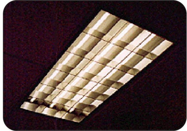
New fluorescent lighting fixtures that incorporate T-8 lamps, electronic ballasts, and good reflectors are key to better lighting at lower cost.
