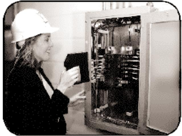
Infrared thermography can quickly identify electrical power system problems and should be included in a proactive maintenance program.
