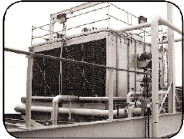
Cooling towers, which are usually components of large HVAC systems, can be made more efficient by controlling their operation times and by retrofitting their motors with variable frequency drives.
