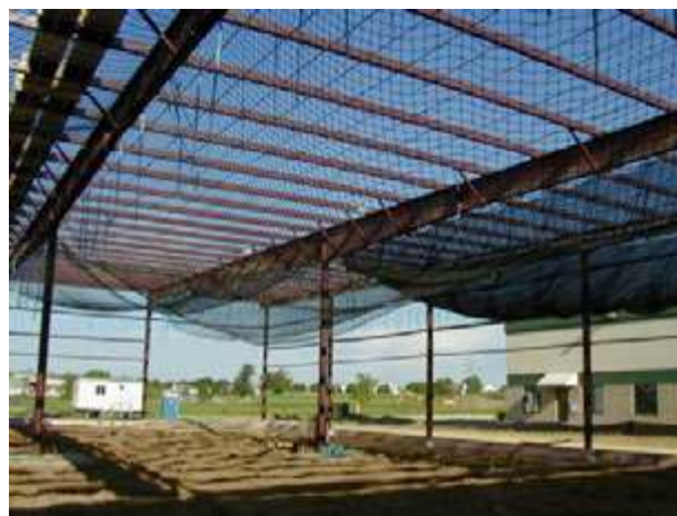
Safety nets used in construction sites.
