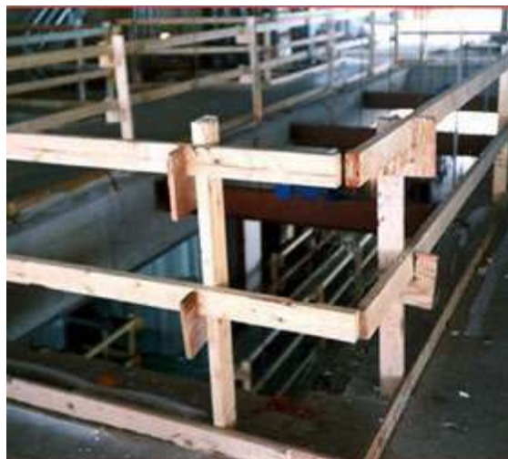
Properly installed guardrail system.
