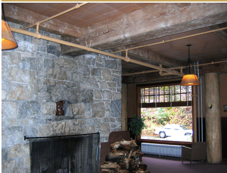
Above: Concealed sprinkler pipe with white sidewall heads have a minimal visual impact on this important historic interior. Below: Exposed sprinkler system in a building where concealing the components would harm the building's historic fabric and thus not be appropriate.
