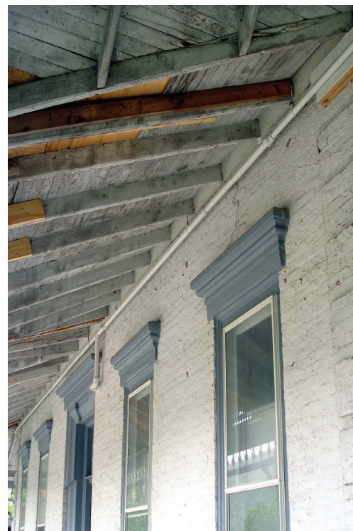
Example of a dry sprinkler sub-zone on the front porch of a historic building in Bellefonte, Pennsylvania. The part of the system that is outside contains compressed air—not water—in the pipes. When these sprinkler heads are activated, the air will escape out of the system, allowing water to flow. The portions of the system that are inside the building where temperatures are above freezing use “wet” pipes.
