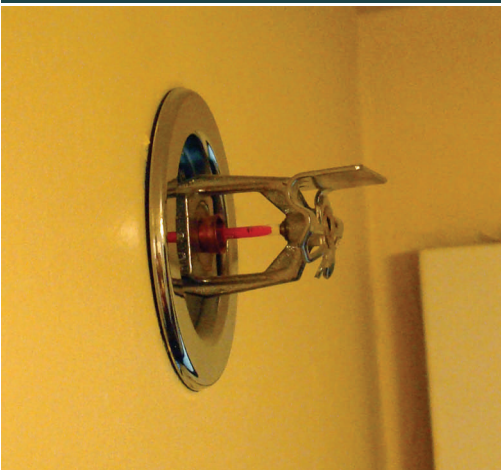
Sidewall Sprinkler Head
