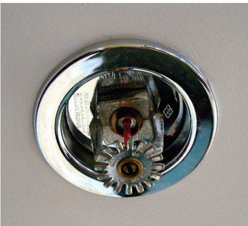
Pendent Sprinkler Head
