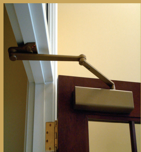
Automatic door closers help reduce the spread of fire through a building and maintain a safe exit route for its occupants. Fire doors are held open by electromagnetic devices that will release and close the doors when the fire alarm activates.
