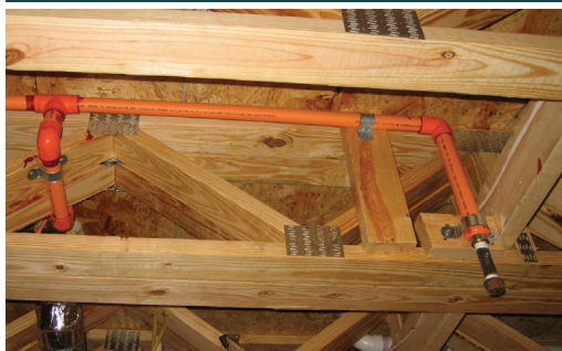
Above: Pendant sprinkler head being fed from both sides by flexible PEX tubing. Below: CPVC
