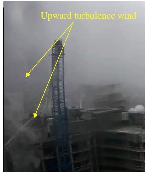
b) Upward turbulence wind detected right after counterweight blocks hit the building
