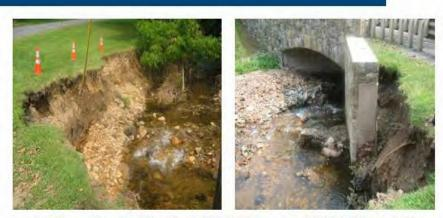
Rt 202 over Branch of Mine Brook, MP 35.42, Structure # 1809153, Bernardsville Boro. Somerset Co, washout & undermining
