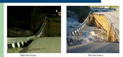
Rt 287 at Rockaway River, NB, MP 44.4, Boonton Twp, Morris Co, 140' x18' x32', right shoulder eroded & wash-out due to abutting Rockaway River size & force
