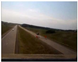
FIGURE 21 Vehicle goes airborne after hitting a heat-buckling site on State Highway 29 Chippewa Falls, Wisconsin, in 2012 (*Courtesy*: Theresa L. Reich).
