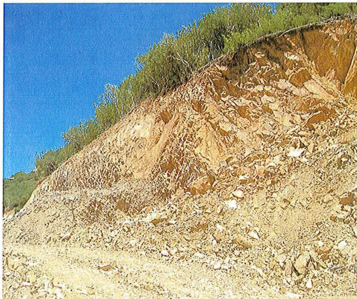
Figure 18. Upper Portion of the Collapsed Surface (South), Looking Toward South.
