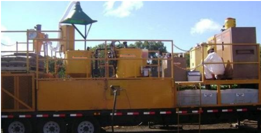
Figure 3.8: Grout plant with two tanks to maintain a continuous supply (courtesy of Applied Foundation Testing).
