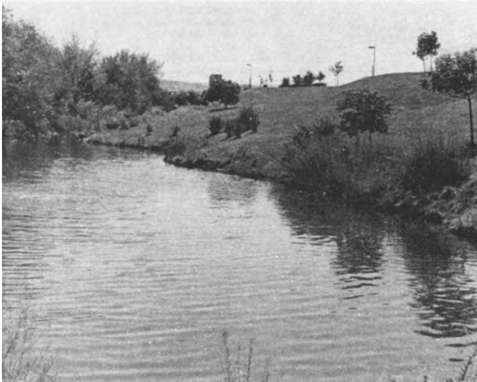
Figure 4-12. Interior flood control collection pond beside levee in Lewiston, Idaho
