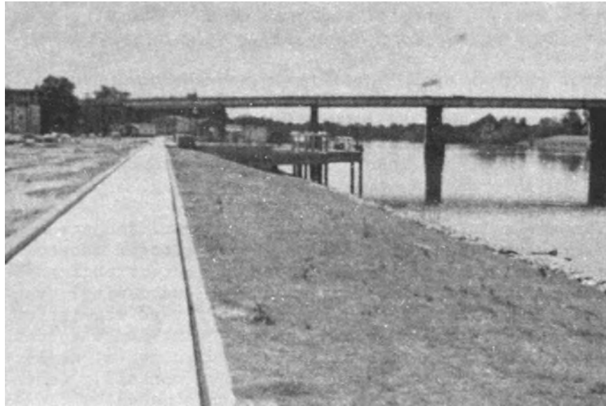
a. Floodwall in the collapsed position
