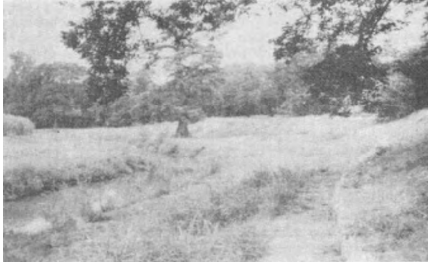
Figure 4-8. Vegetative lining, San Antonio River flood channel (USAED, Fort Worth). This completed reach contains a subchannel that conveys normal flows. The high-flow berms and banks are vegetated. Note the River Walk (Paseo del Rio) inside the flood channel
