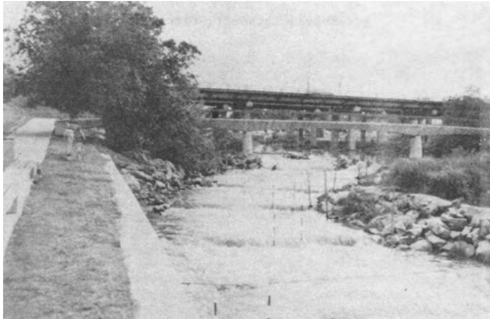
Figure 4-18. Confluence Park boat chute, South Platte River, Denver. A series of 12 pools and weirs drop 10 feet over a run of 330 feet.
