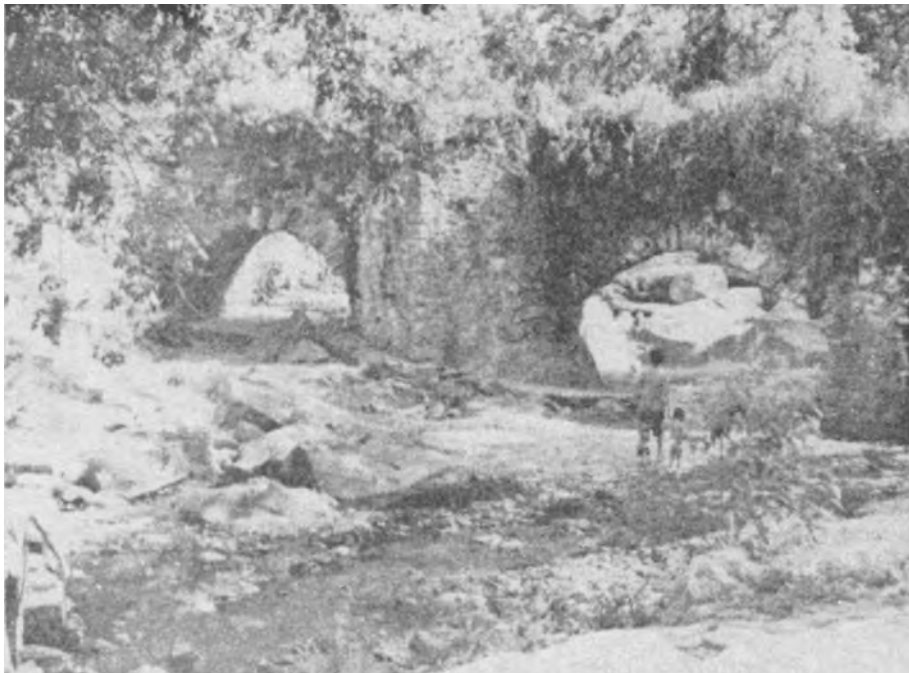
b. Espada Aqueduct in 1977
