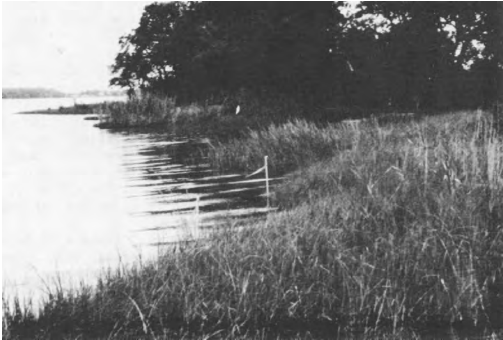
a. Vegetative erosion control project (Maryland)
