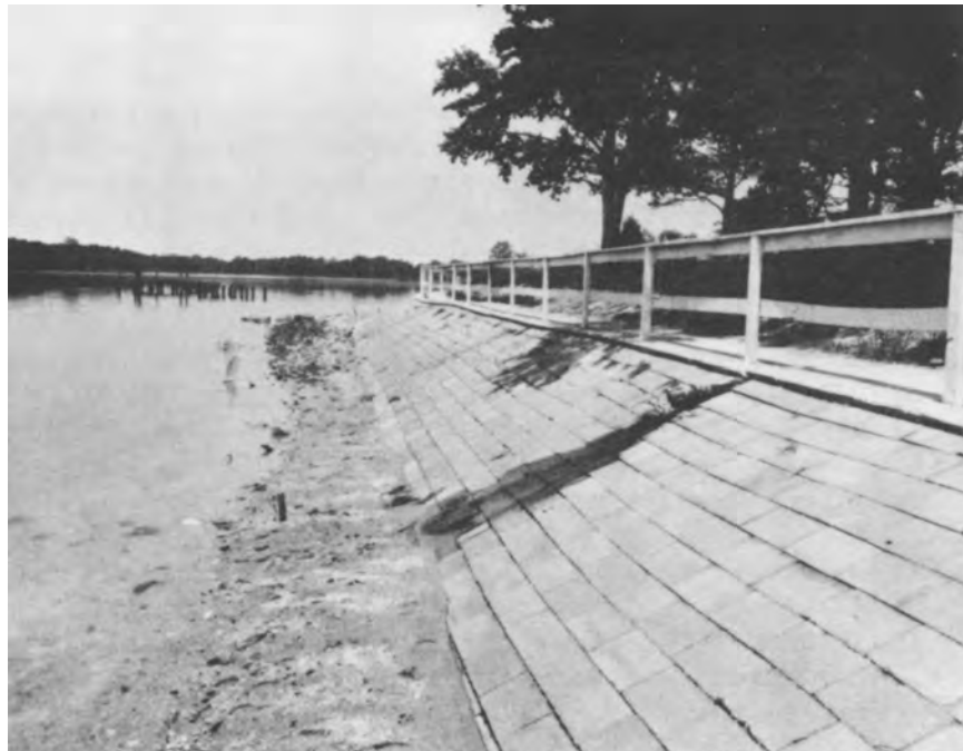
b. Erosion control structure (Maryland)
