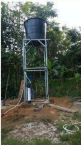
Fig. 1: Install water storage tanks with RFU*
