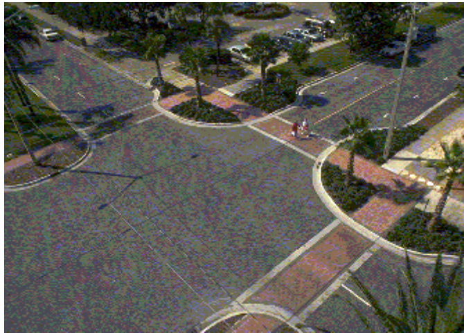
Figure 3. Bulbouts shorten crossing distances for pedestrians, improve sight distances, and may slow vehicle speeds.
