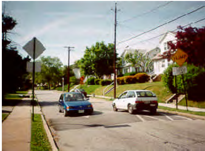
Figure 1. Two vehicles slow down as they pass over a speed hump.
