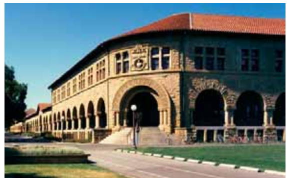
Figure 8-25: Stanford University Quad Corner Buildings. The four very similar corner buildings were also seismically strengthened over a 40-year period. Substantially different techniques evolved due to growing recognition of the historic value of the entire Quad. The first corner was “gutted” in 1962 and an entire new structure built inside with two added floors. The second corner was done in 1977 and was also gutted, but the original floor levels were maintained and interior finishes were similar to the original. The last two corners, repaired and retrofitted following the 1989 Loma Prieta earthquake, were strengthened with interior concrete shear walls, while the bulk of the interior construction was maintained, including the wood floors and heavy timber roofs.
