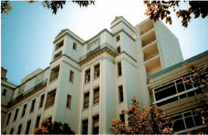
Figure 8-12: External towers were added to strengthen this building from the outside. The new tower is the element at center-left of the figure. The retrofit scheme for this building is discussed in detail in Figure 8-9.
