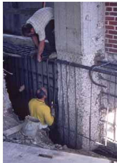
Figure 8-11: Retrofit activities inside buildings are most often not surgical or delicate. Here work on a new foundation for a shear wall is prepared for casting.
