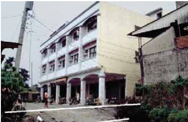
Figure 2-5: This building near Juahan, in Taiwan, was lifted several feet by the fault. Fault rupture runs just near the side of the building, down the alley. The white lines highlight the offset ground surface. There was no apparent damage to the building.
