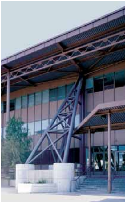
Figure 8-17: A modern exterior buttress used for seismic strengthening.
