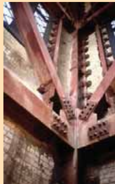
Figure C: Steel space frame inserted within tower
