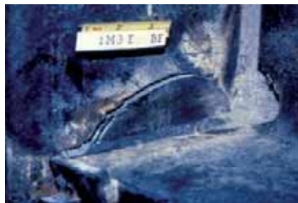
Figure 8-3: An example of a recently designed building with seismic deficiencies not understood at the time of design. In this case, the deficiency was “pre-Northridge” moment-frame connections, which proved to be extremely brittle and unsatisfactory. Hundreds, if not thousands, of these buildings were designed and built in the two decades before the Northridge earthquake (1994).
