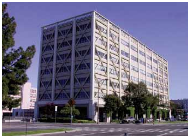
Figure 8-15: Renovation and retrofit of a concrete warehouse structure by removing the exterior wall, inserting steel braces and window wall, and adding construction on the inside of the building.
