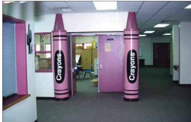
Figure 9-2: Limited nonstructural damage at Landers Elementary.
