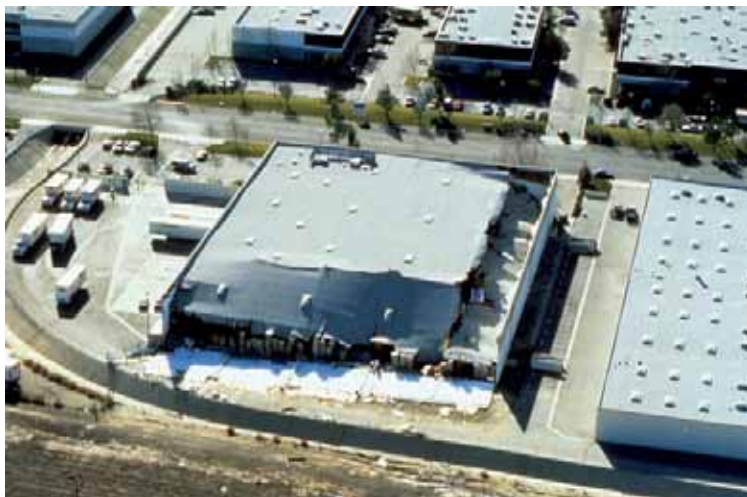
Figure 8-6: A tilt-up damaged in 1994. Despite suspicions that the code-required roof-to-wall ties were inadequate, it took several code cycles and incremental increases in requirements to obtain adequate code provision. Thousands of tilt-ups with inadequate connections exist in the West, although several jurisdictions are actively requiring retrofits.
