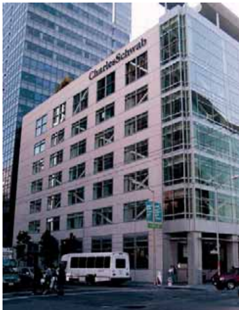
Figure 8-15: Renovation and retrofit of a concrete warehouse structure by removing the exterior wall, inserting steel braces and window wall, and adding construction on the inside of the building.
