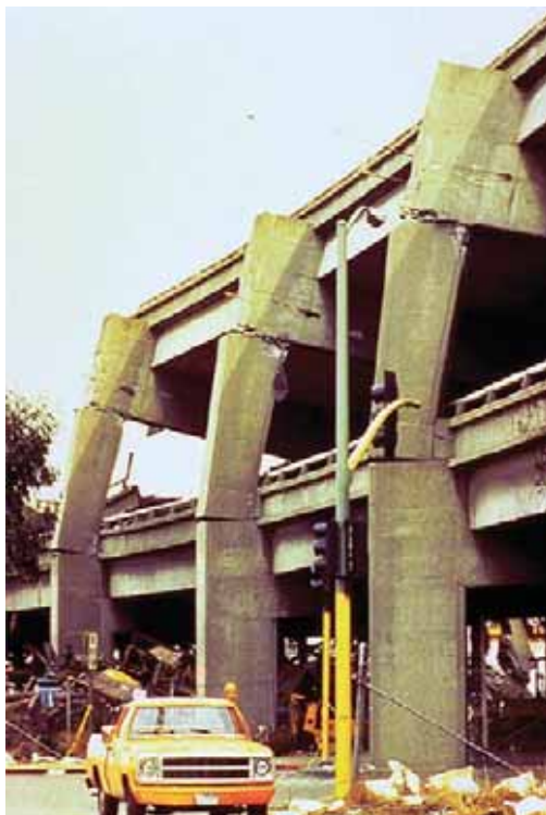
Figure 6-6: San Francisco, 1989, elevated highway support bents, an example of failure of engineered structures.
