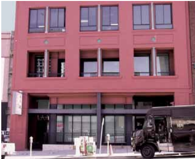
Figure 8-14: Examples of steel moment frames in similar commercial retrofits. Right: Note the large white column and double beam arrangement. Left: The moment frame is placed against the wall of the recess. The first floor columns are gray and the balance is pink. The frame can be seen on both the first and second floors.
