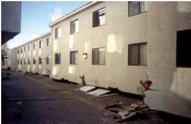
Figure 8-5: A tuck-under similar to Figure 8-4, but much more modern and designed at a time when the weakness of the parking level was more understood. In this case, the detailing of the small wood shear walls at that level was poor. This practice created another set of deficient “existing” buildings.
