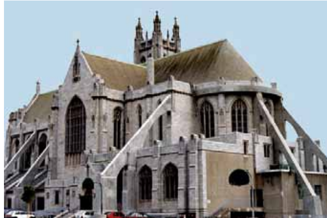
Figure 8-22: St. Dominic's Church in San Francisco was seismically retrofitted using exterior buttresses.
