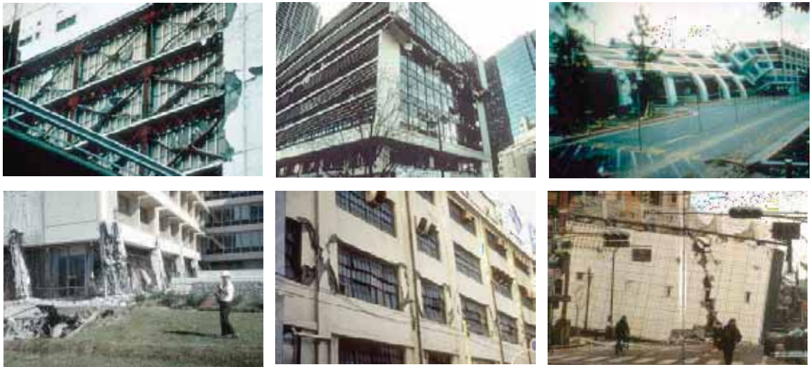
Figure 7-12: Examples of typical earthquake damage.
