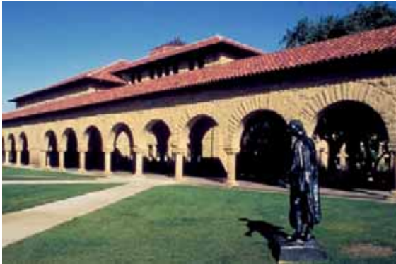
Figure 8-24: Original Quad arcades, Stanford University. The Quad, approximately 850 feet by 950 feet in plan, is surrounded by a covered arcade. Modern seismic retrofits have taken place over a 40-year period, with evolving techniques. Final sections were completed by removal of the interior wythe of sandstone, installation of reinforced concrete core, and reinstallation of the interior blocks, which were reduced in thickness. Due to environmental decay of many of the sandstone columns, additional seismic resistance was obtained in many locations by installation of precast concrete replicas that formed a part of a continuous vertical reinforced concrete member.
