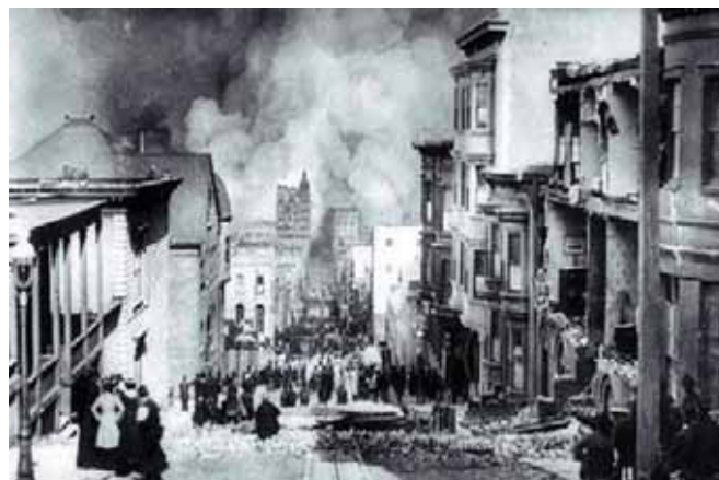
Figure 6-1: San Francisco 1906, fire and earthquake damage.
