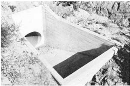
Figure 7-7. Type 4 inlet concrete transition. P-328-701-9300
