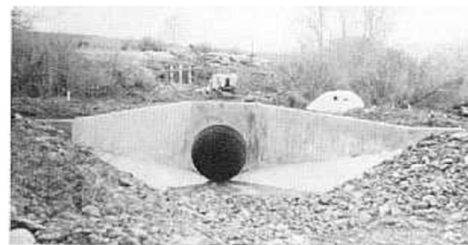
Figure 7-1. Type 1 concrete transition, P33-D-25693
