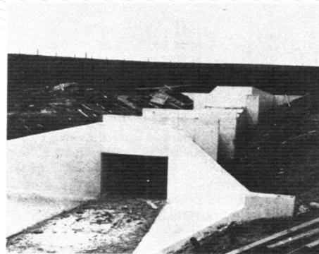
Figure 4-21. Concrete box culvert with concrete percolation collars. P328-701-3743
