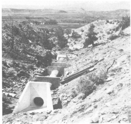
Figure 4-19. Culvert, constructed prior to construction of canal. PS14-417-366
